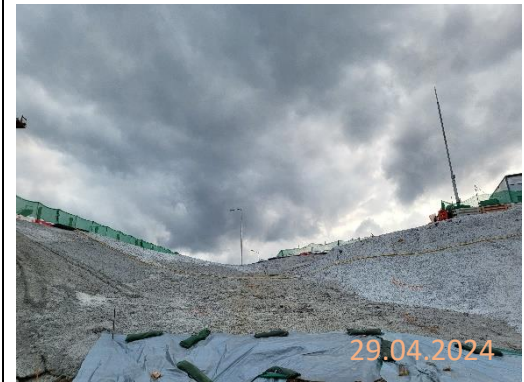
By subcontractor at KNP site
