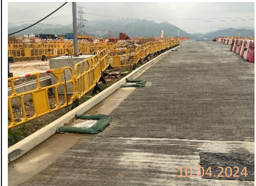
By main contractor at KNP site
