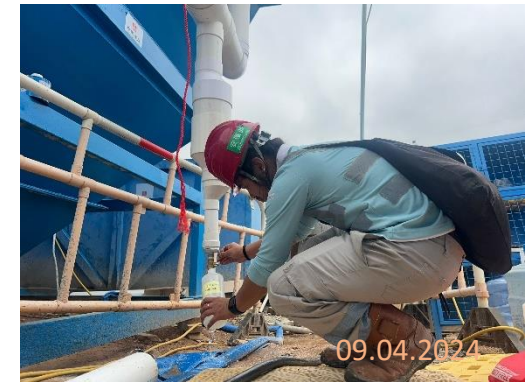
By main contractor at KNP site
