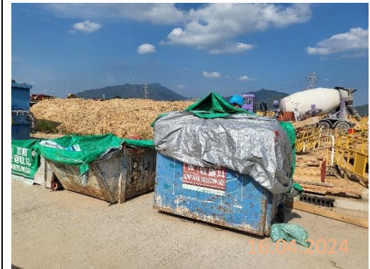
By main contractor at KNP site
