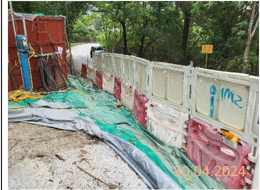
By main contractor at KNP site
