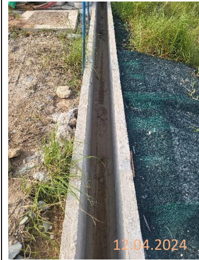
By main contractor at KNP site
