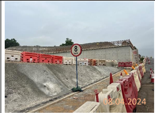
By main contractor at KNP site
