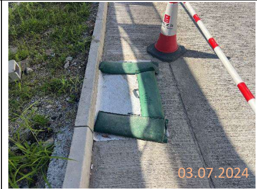
By main contractor at KNP site
