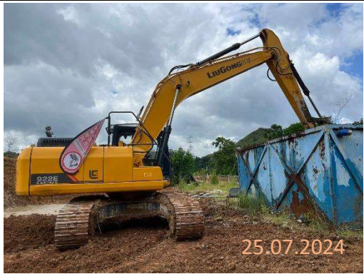
By main contractor at KNP site
