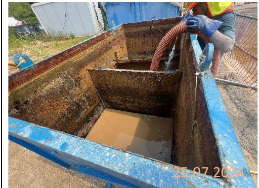
By main contractor at KNP site
