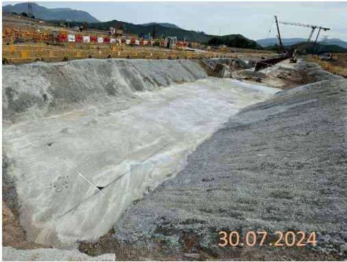
By subcontractor at KNP site
