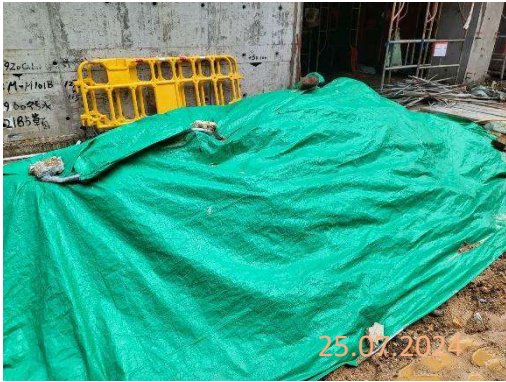
By subcontractor at KNP site
