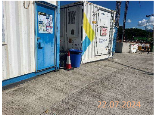
By main contractor at KNP site
