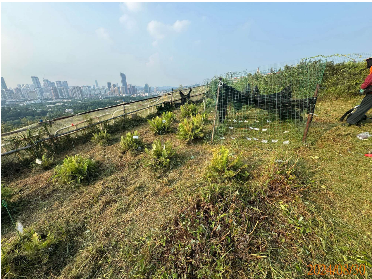
Replacement of protection fence (2)
