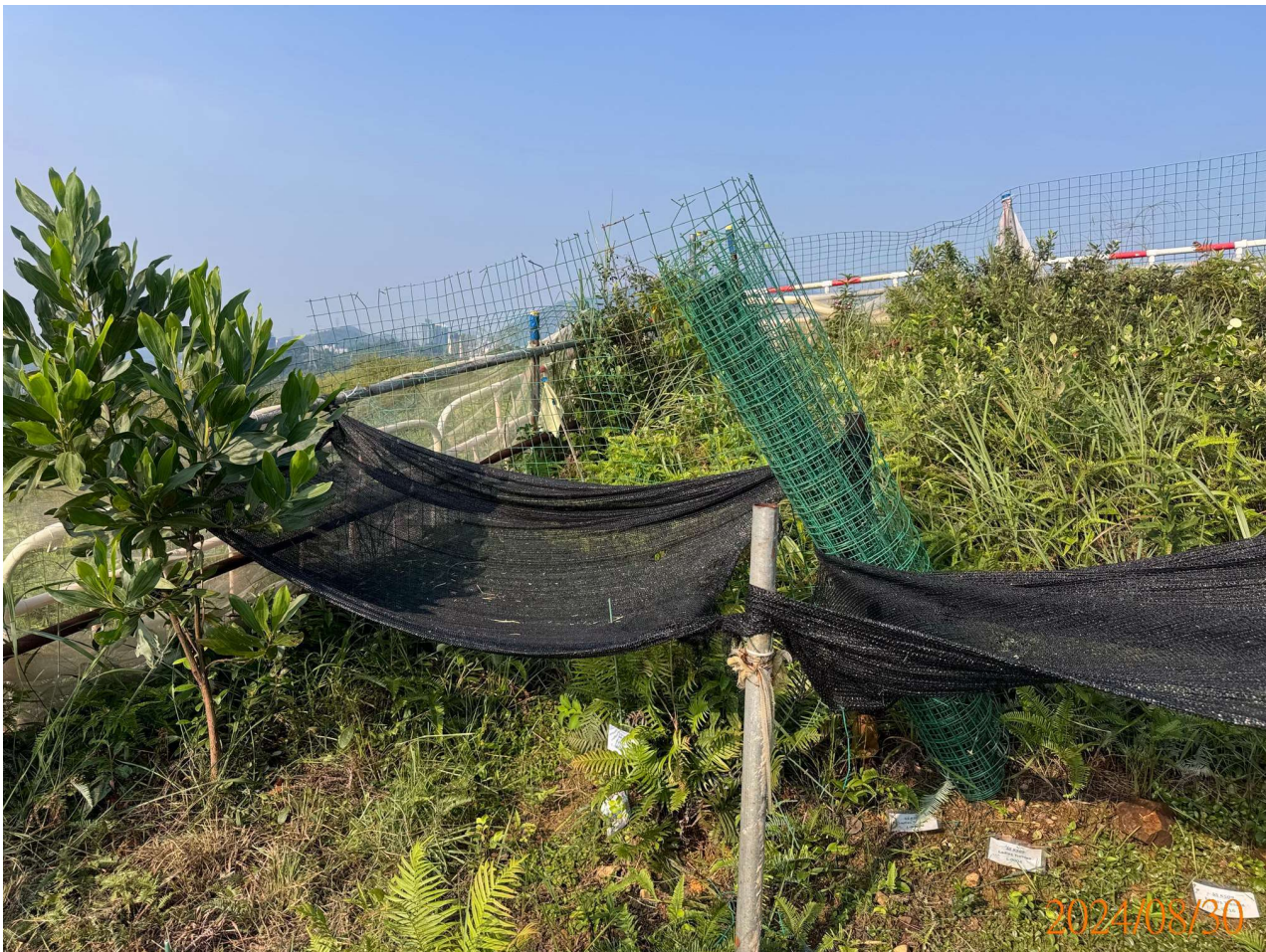
Replacement of protection fence (1)
