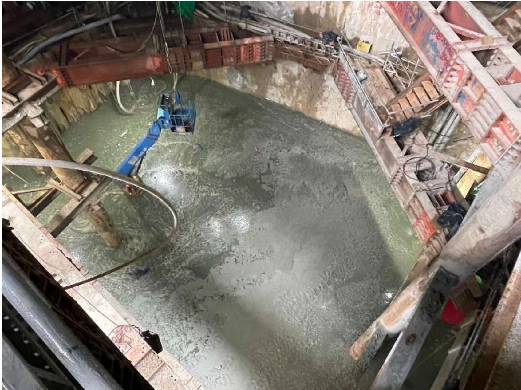
Remark 3: On-site photo
