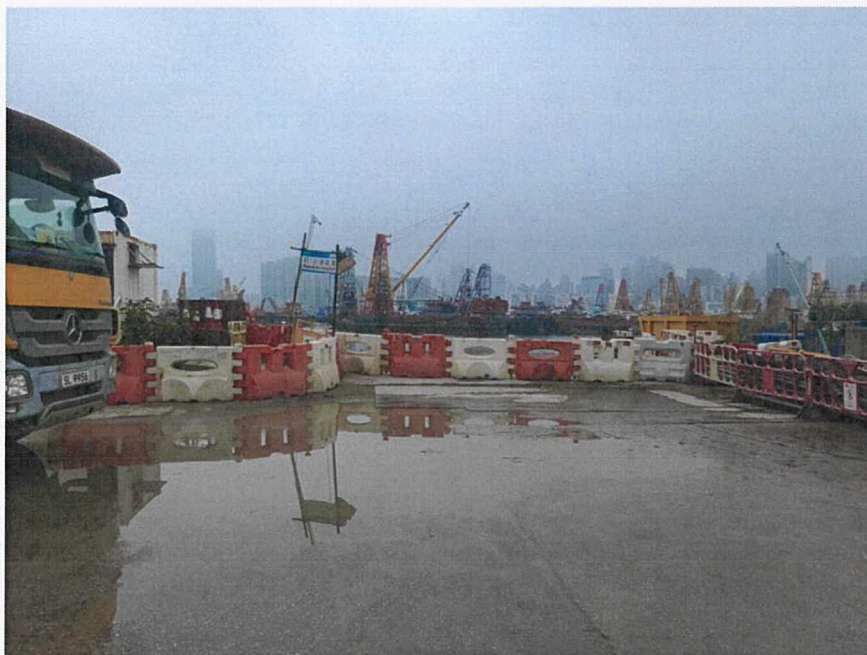
Photo 3.1 (Kai Tak Barging Facility - Gammon Construction Limited.)
