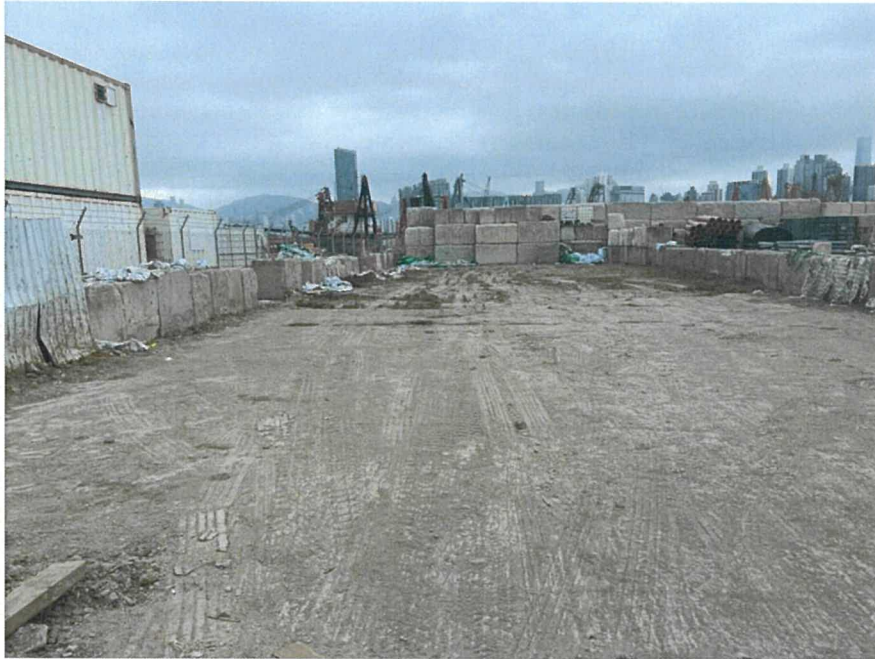
Photo 3.7 (Kai Tak Barging Facility - Build King – SK Ecoplant JV)
