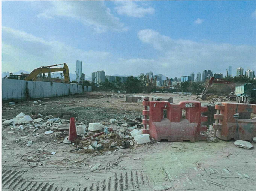
Photo 3.5 (Kai Tak Barging Facility - Hip Hing Construction Limited)
