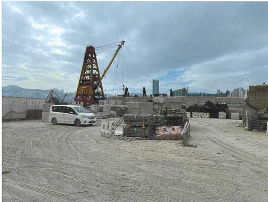
Photo 3.3 (Kai Tak Barging Facility - Bouygues Travaux Publics)
