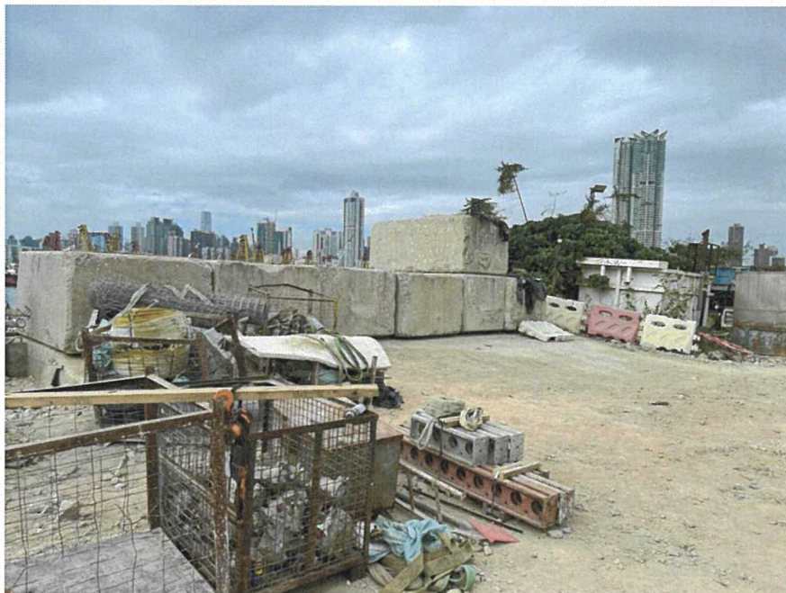
Photo 3.4 (Kai Tak Barging Facility - Bouygues Travaux Publics )
