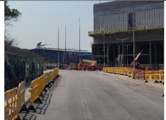
Reinstatement of access road
