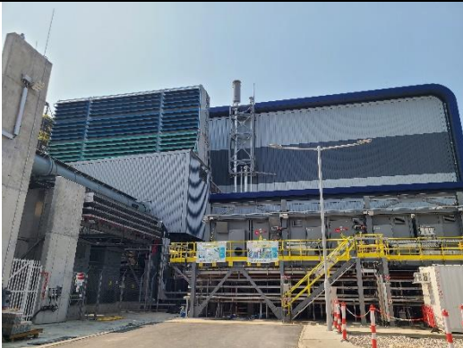
Turbine Hall (Exterior)
