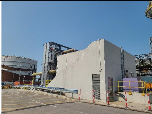
Cooling Water Discharge Facility
