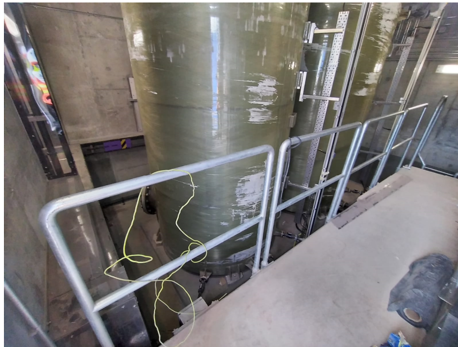
Fluorosilicic Acid Storage Bund
