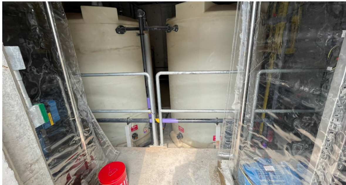
Sodium Hydroxide Bund Area
