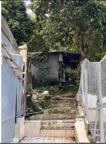
Plate 1 相片 1 – FHT1: Squatter House out of the Northwestern Entrance of the Existing Lam Tei Quarry 現有藍地石礦場西北面入口外的寮屋
