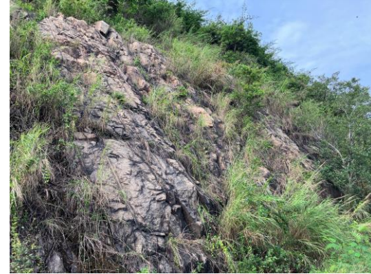
Plantation (Project Site)
