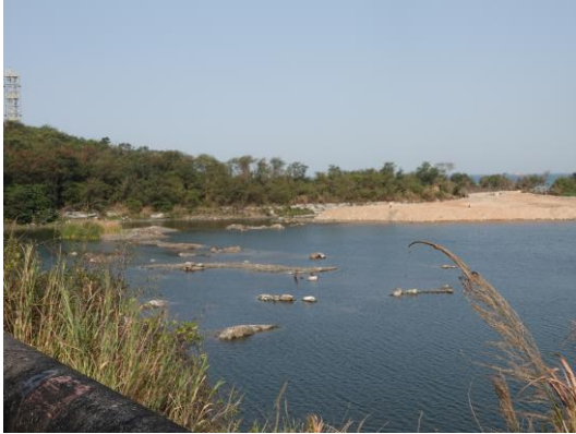
Ash Lagoon (Project Site)
