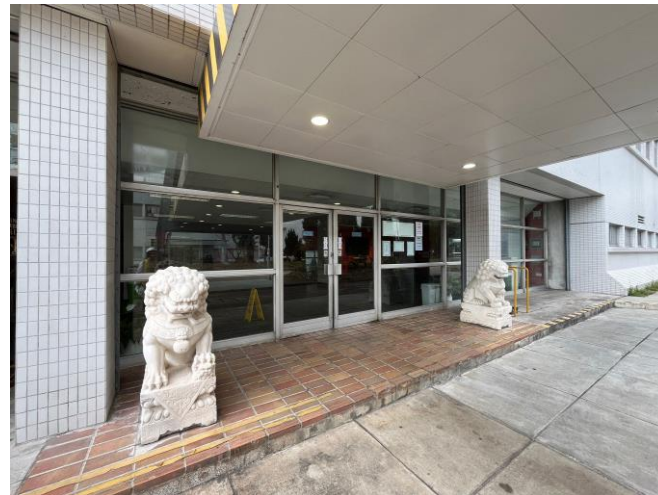
Photo 59: Entrance of the administration building
