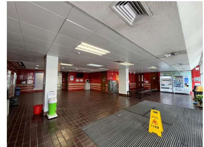
Photo 60: Lobby of the administration building
