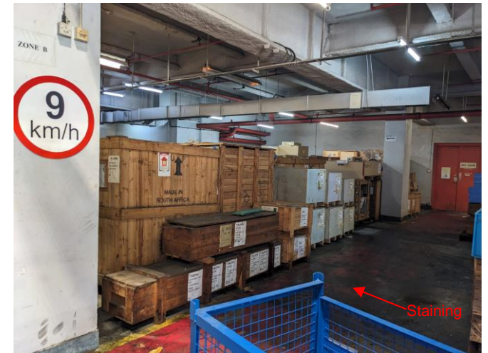
Photo 66: Store area in the control block, workshop and store building
