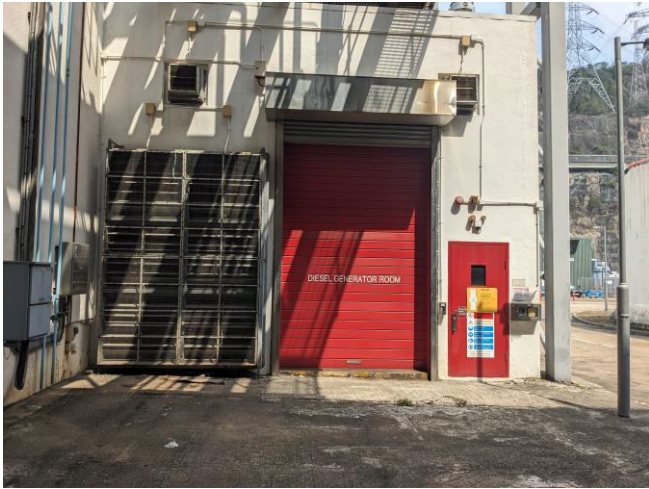
Photo 43: Black start diesel generator room
