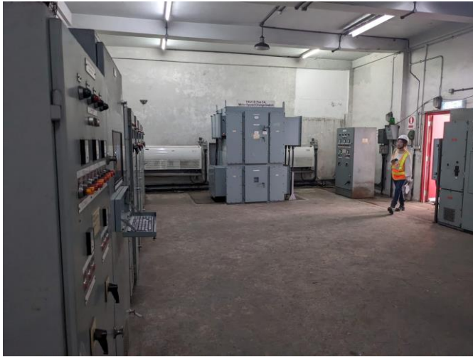
Photo 85: Precipitator Control Building
