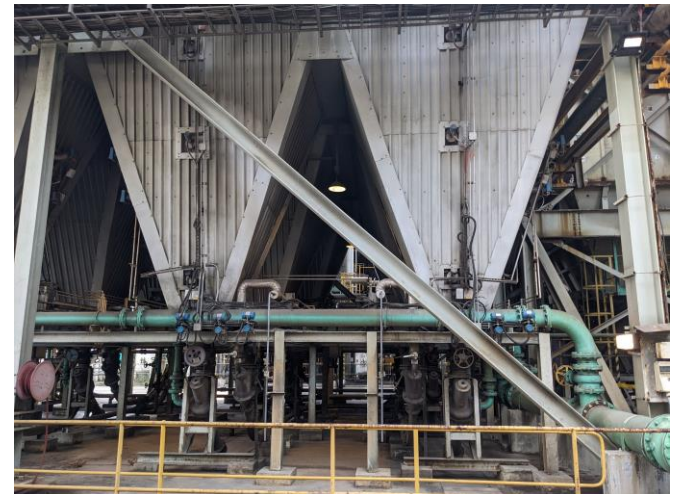
Photo 54: Electrostatic precipitator systems including ash hoppers for fly ash
