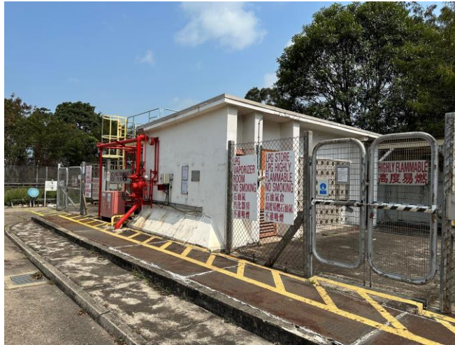
Photo 80: Liquefied Petroleum Gas (LPG) Store
