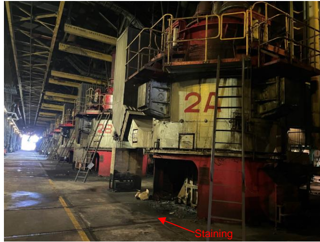
Photo 8: A series of coal grinding mills along CPA Station Building
