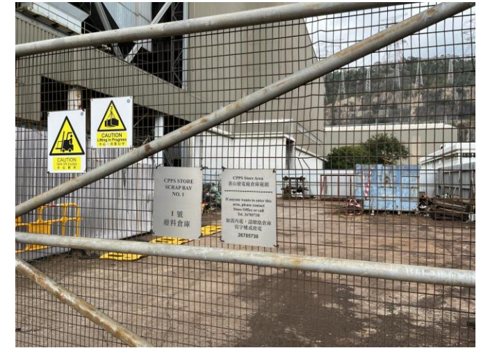
Photo 96: Scrap yard at southeast boundary of the Project site
