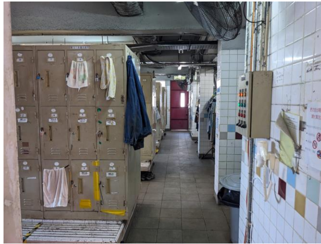
Photo 74: Welfare building for the ash plant workers
