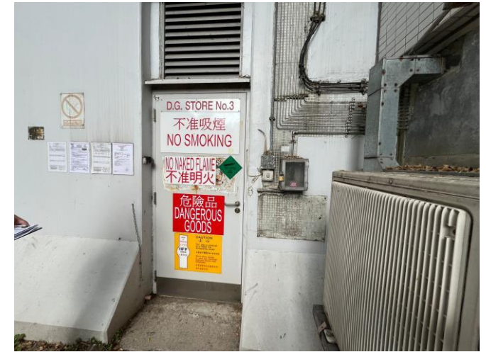
Photo 63: Dangerous goods store No.1 and No.2 in administration building
