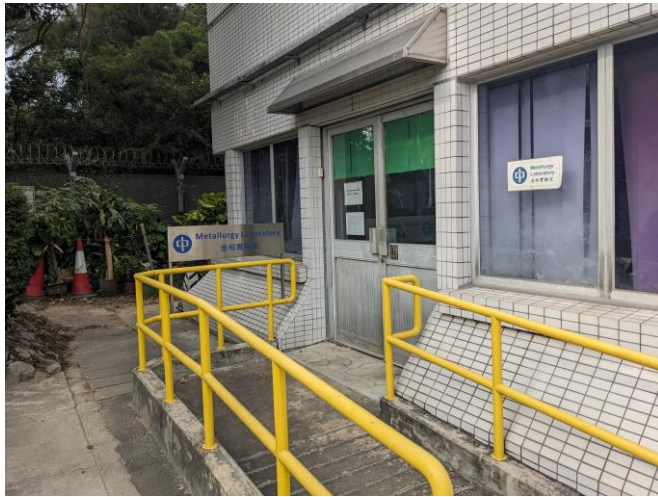
Photo 61: Metallurgy laboratory in administration building
