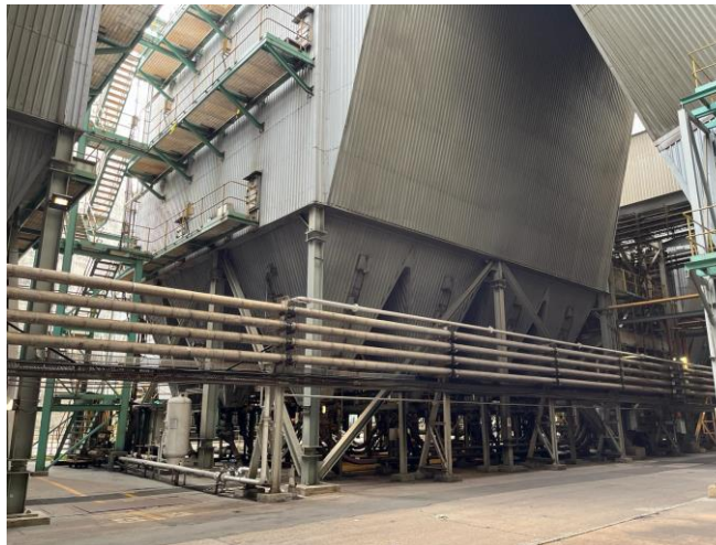
Photo 53: Electrostatic precipitator systems including ash hoppers for fly ash
