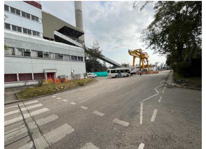
Photo 102: Access road along the northwest of the Project site boundary
