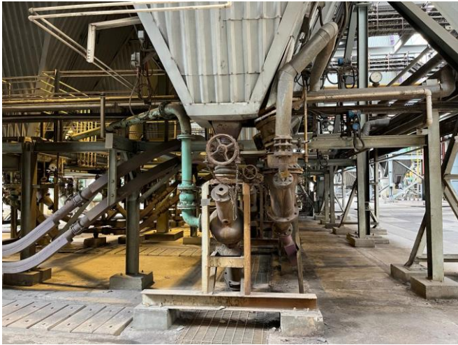
Photo 55: Bottom of electrostatic precipitator ash hopper structures
