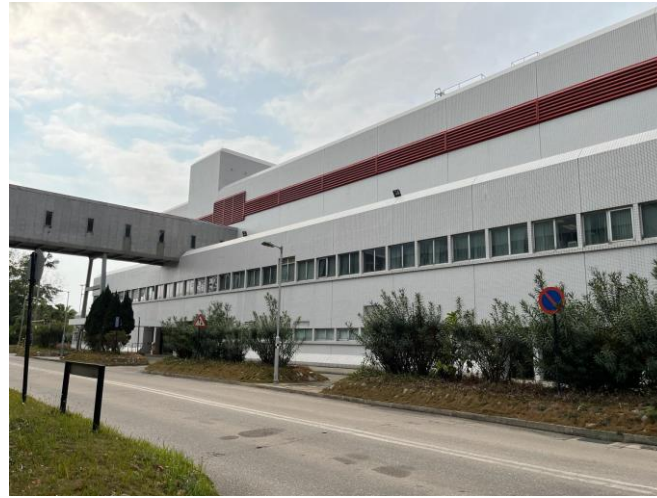
Photo 101: Planter and access road outside the administration building
