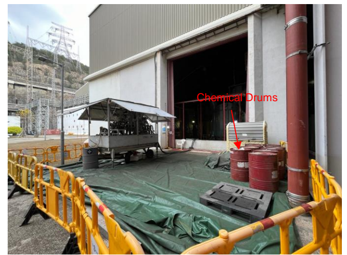
Photo 42: Transformer maintenance area at units A4
