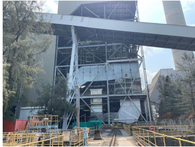
Photo 68: Ash pits area
