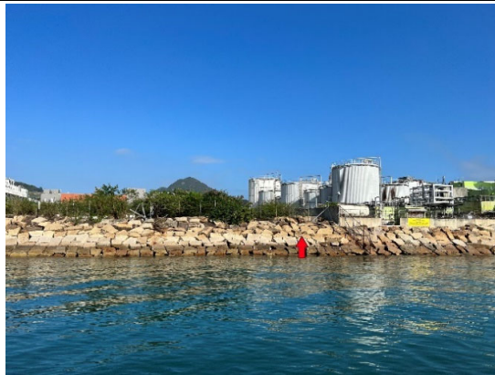
Figure 1.2b Photographs of the Landing Site and its Surroundings at TKOIE
