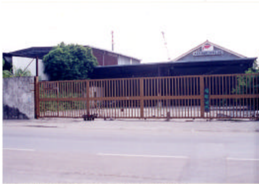
9 YMTL 26 VACANTED WAREHOUSE
