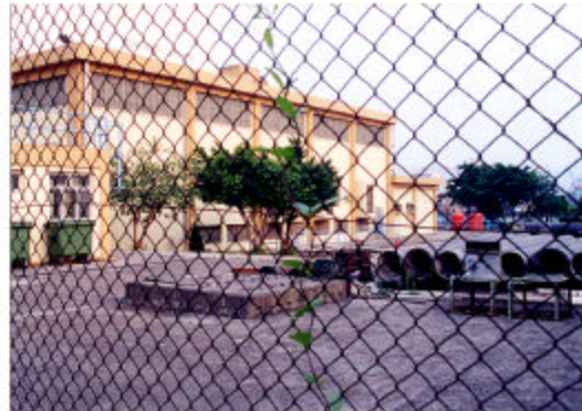
2 SALT WATER PUMPING STATION
