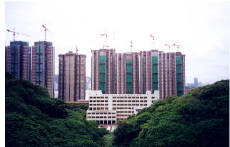
12. VIEW FROM PIK WAN ROAD NEAR HONG PAK COURT
