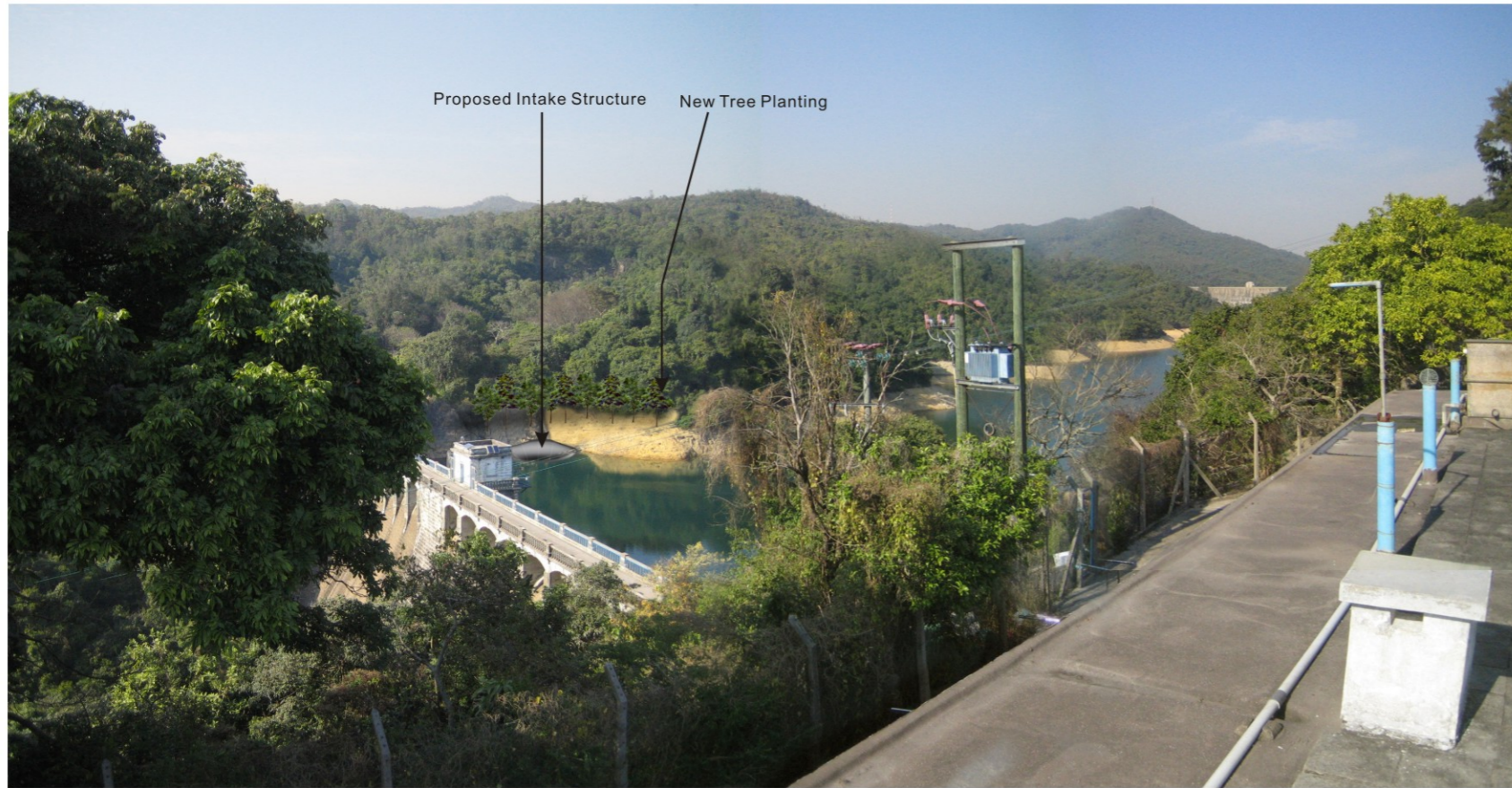
Operation Phase - Day 1 with mitigation measures newly implemented
