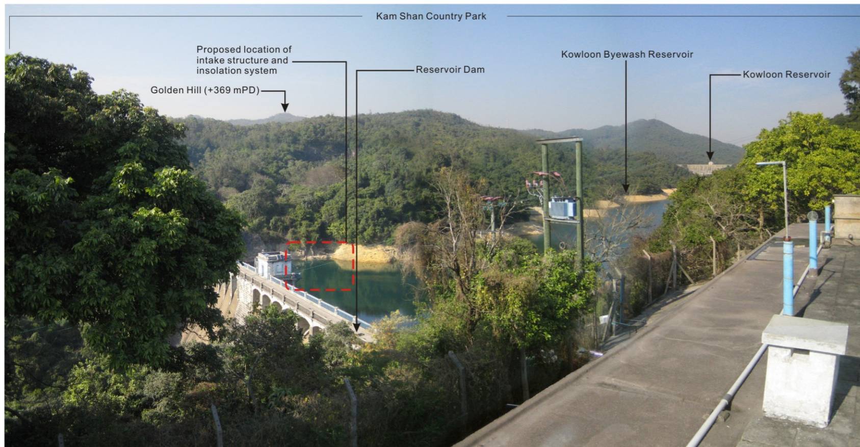
View from Abandoned WSD Staff Quarters (Existing Situation)
