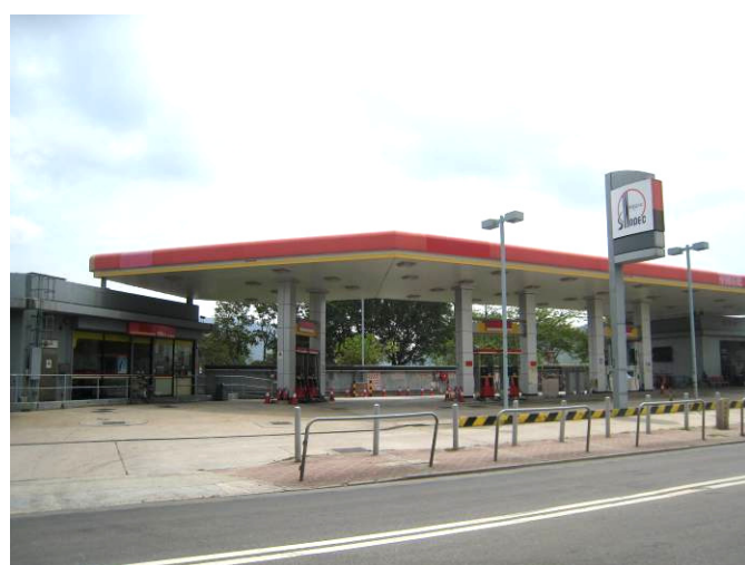
Photo 18. Petrol & LPG filling station located near the Kam Tin Clinic
