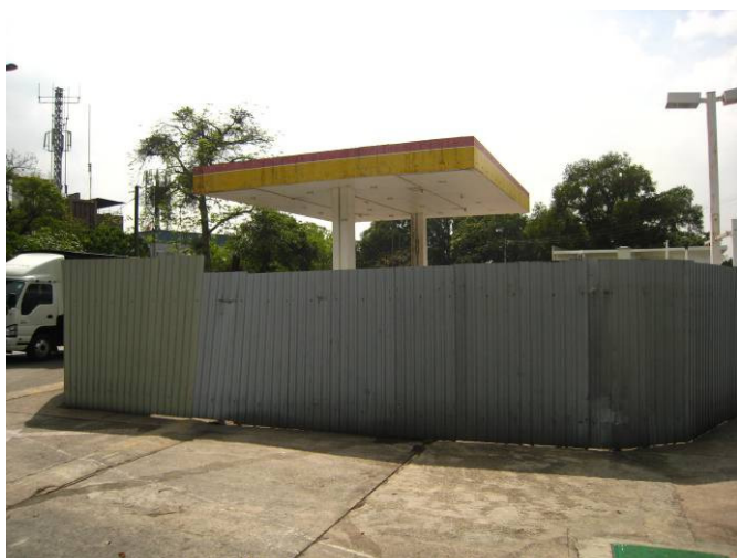
Photo 5. Vacant petrol station located near the Sheung Tsuen Park
