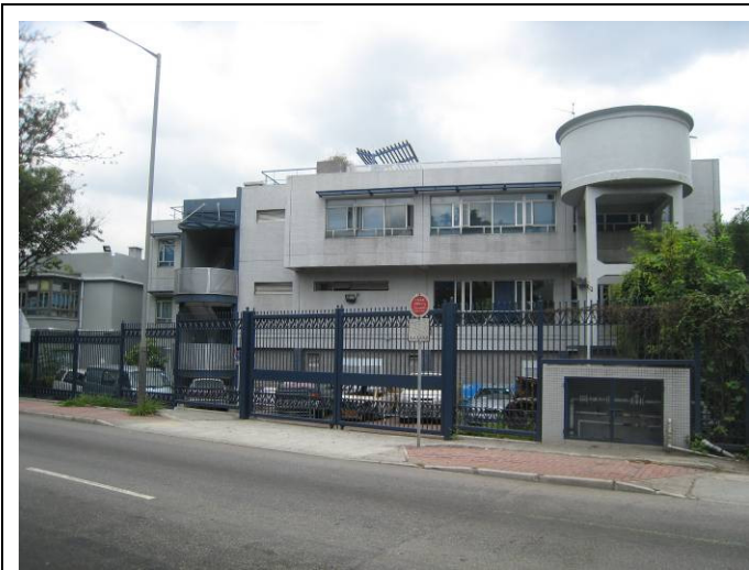
Photo 13. Pat Heung Division Police Station located next to Kam Tin Road
