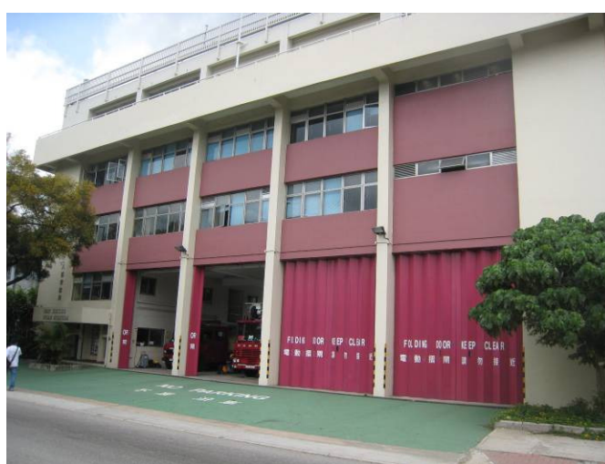
Photo 12. Pat Heung Fire Station located next to Kam Tin Road
