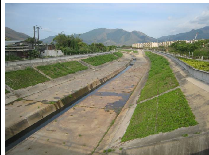
Photo 9. Kam Tin River Channel
