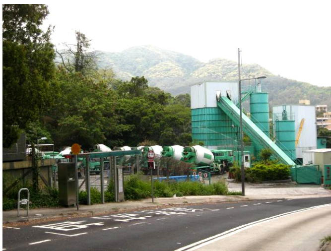
Photo 3. Concrete batching plant located next to Lam Kam Road
