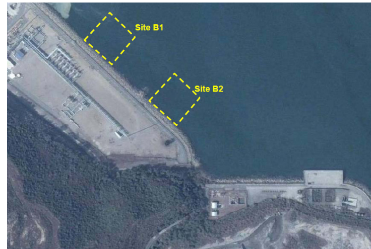
Sites B1 and B2 - Reclamation adjacent to the existing GRS
