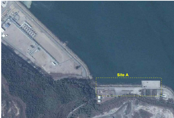
Site A - Western side of the West Ash Lagoon
