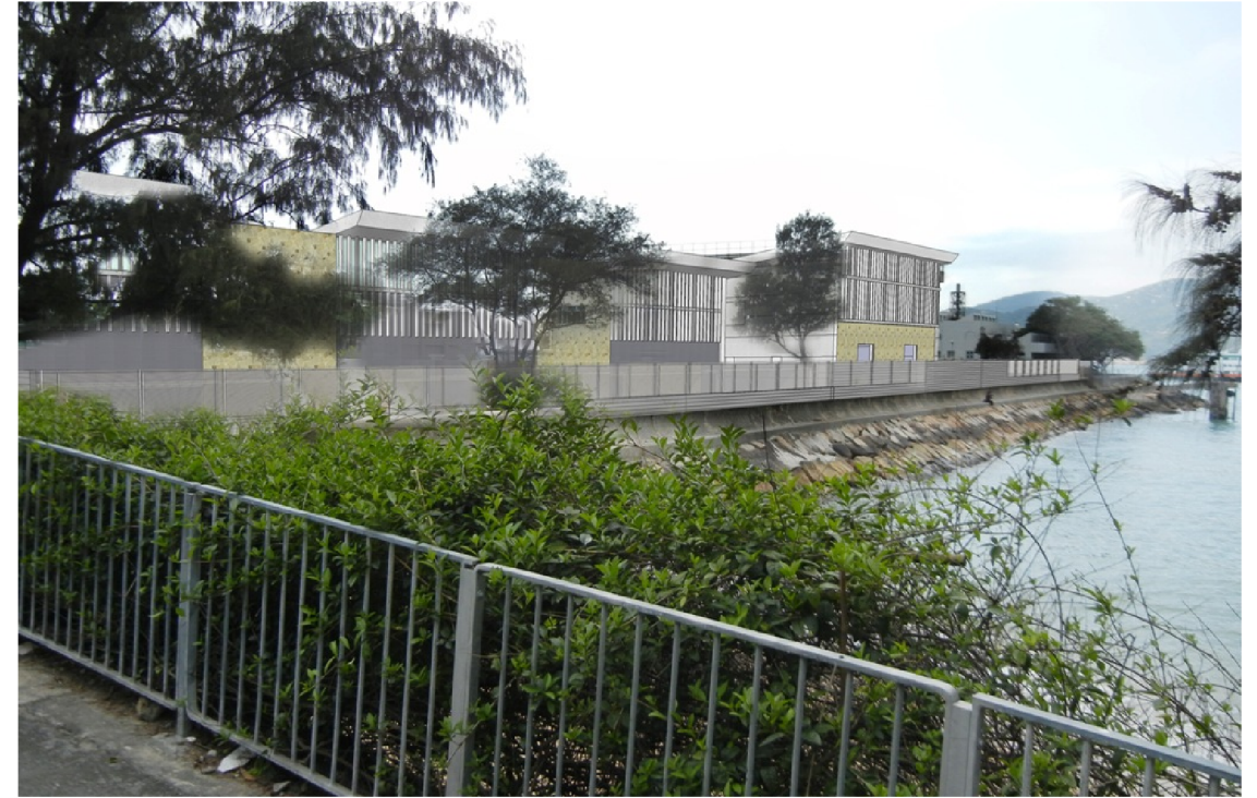
View of the Proposed Cheung Chau STW Upgrading - without visual mitigation measures
