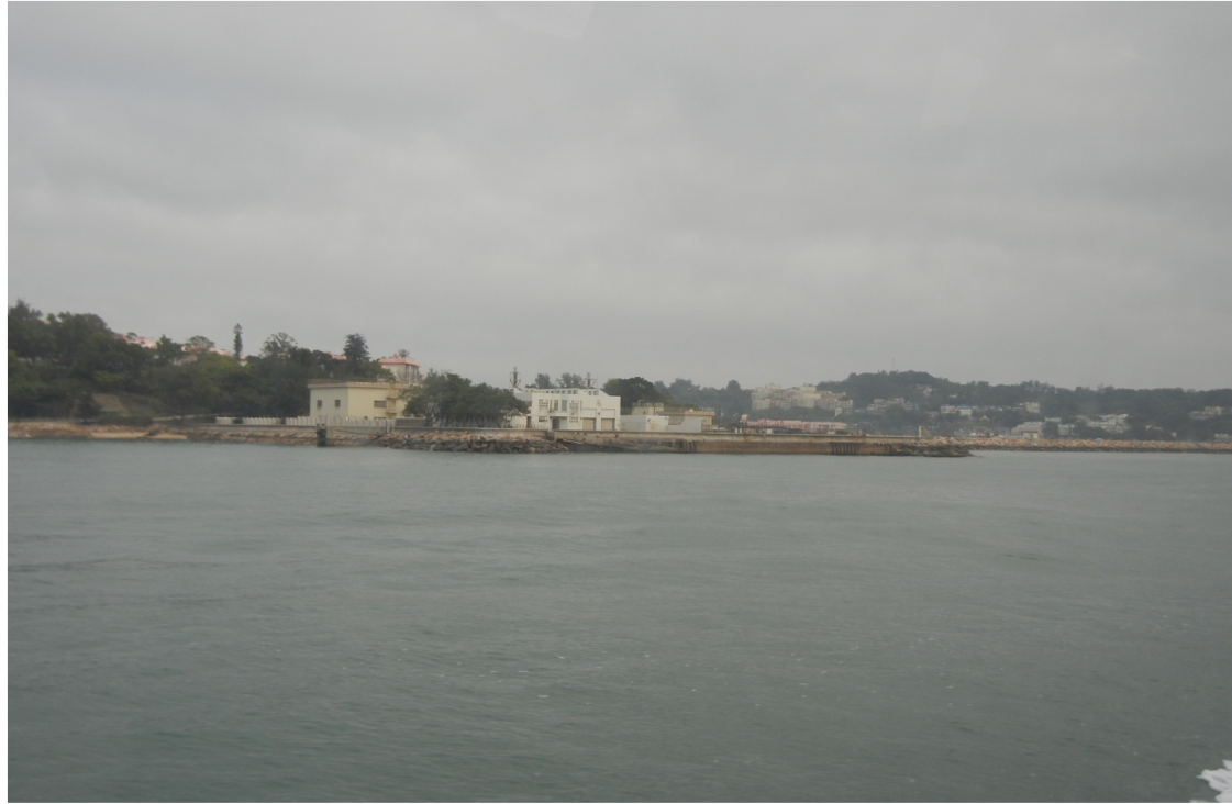
Existing View of the Cheung Chau STW
