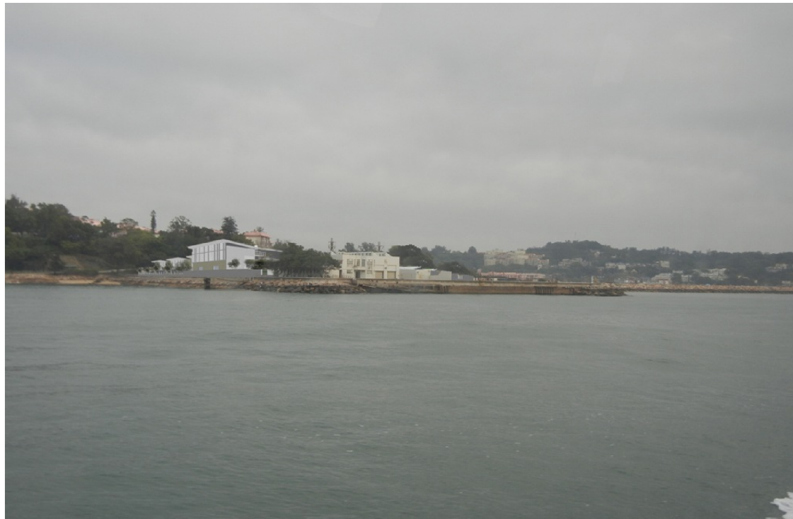
View of the Proposed Cheung Chau STW Upgrading - with visual mitigation measures - Day 1
