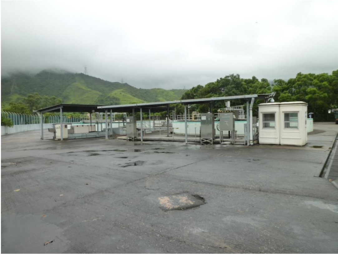
Photo 7 - Existing Sha Tau Kok Sewage Treatment Works
