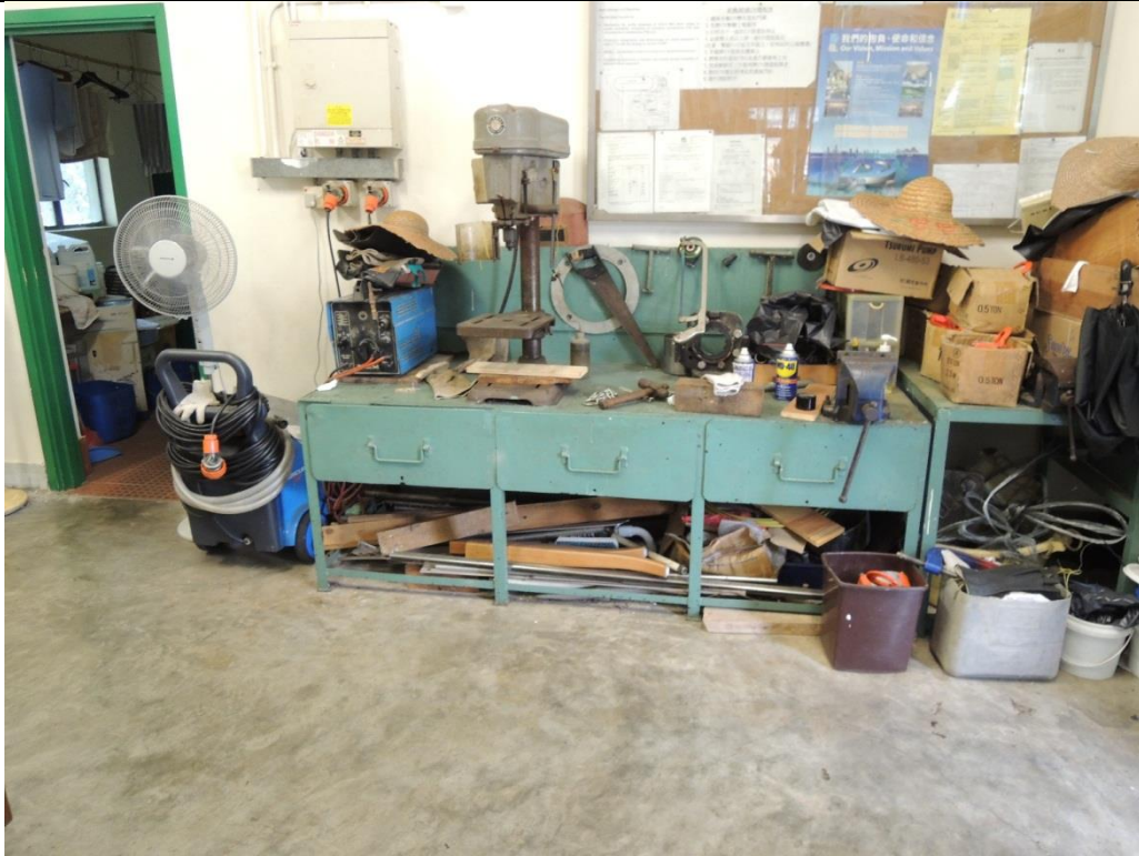
Photo 9 - Workshop of the Existing Sha Tau Kok Sewage Treatment Works (Interior View)
