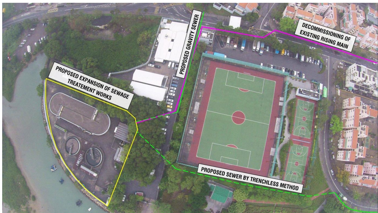
Photo 12 - Bird's Eye View of Existing Sha Tau Kok Sewage Treatment Works
