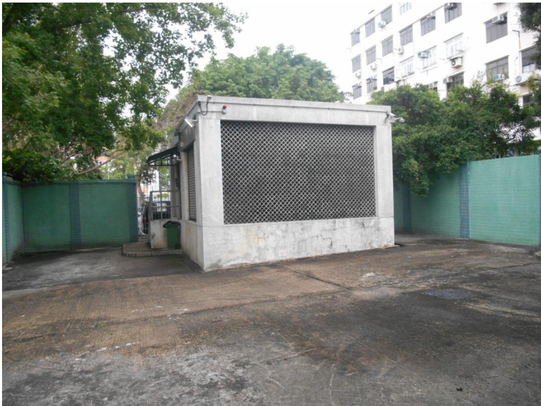
Photo 2 - Existing Sha Tau Kok Sewage Pumping Station at Shun Hing Street
