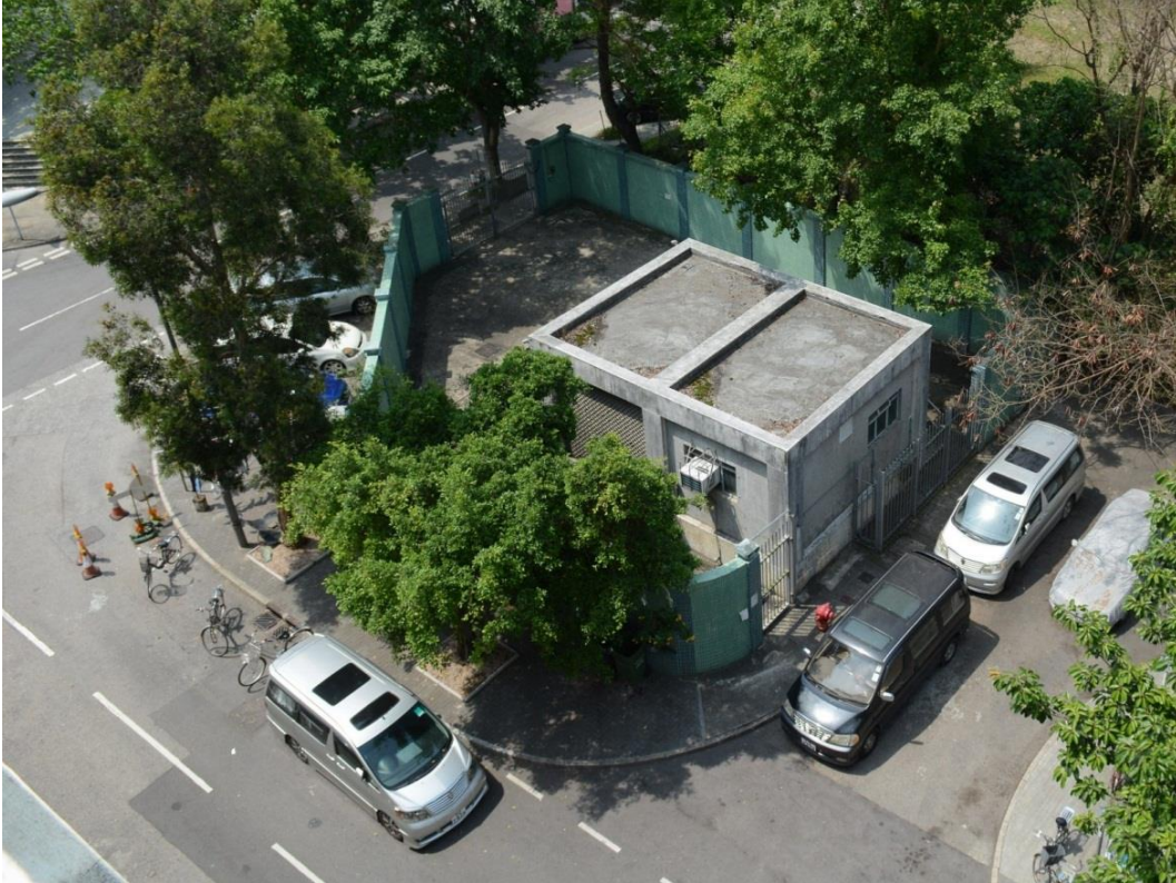
Photo 1 - Bird's Eye View of Existing Sha Tau Kok Sewage Pumping Station at Shun Hing Street
