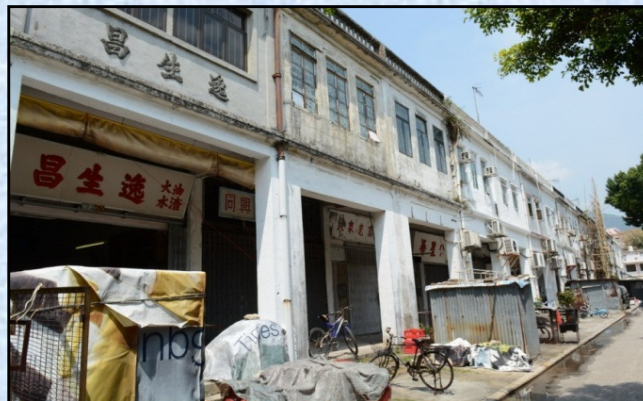
LR8.5 - Shophouses at San Lau Street
