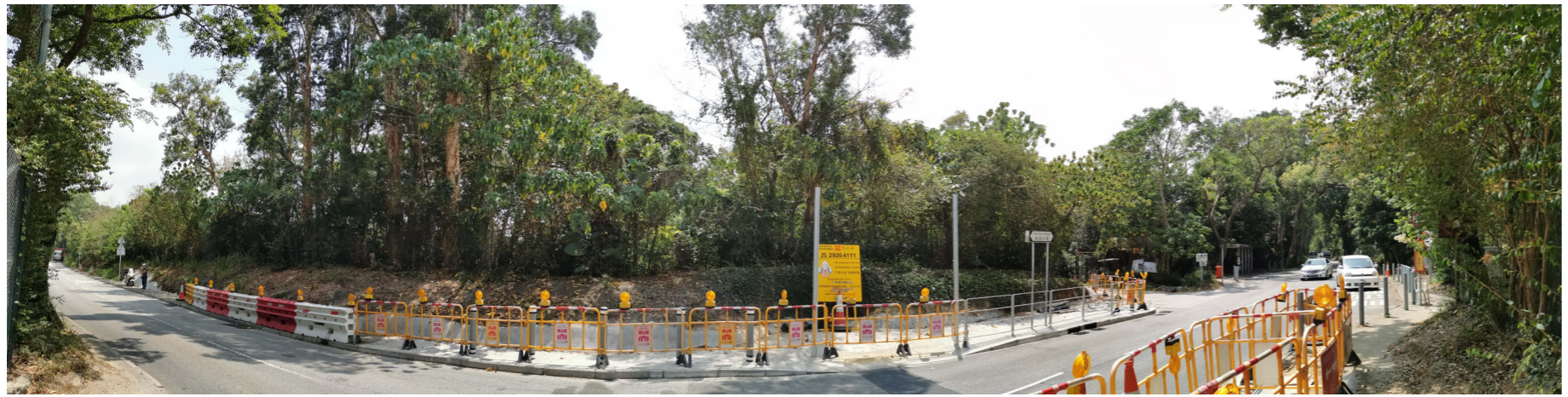
VP13 - FAN KAM ROAD - EXISTING SITE CONDITION
