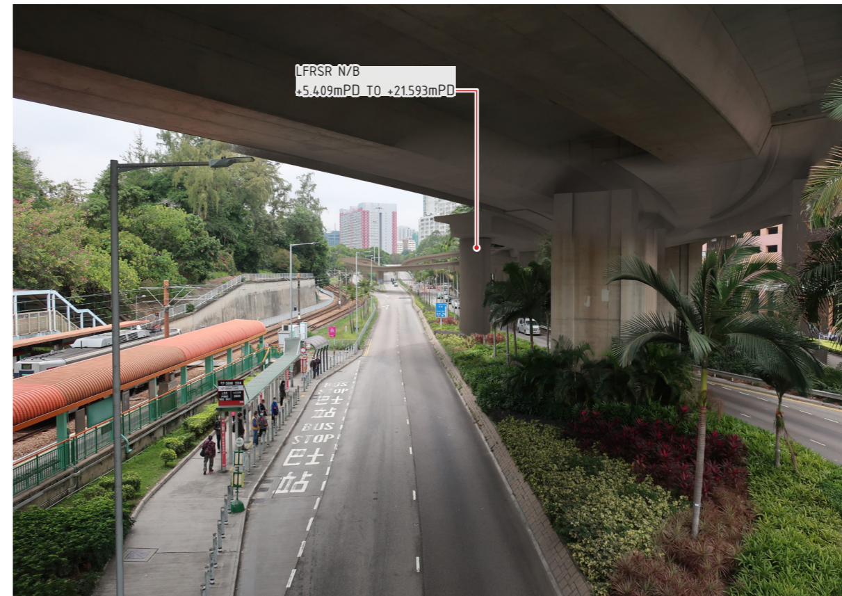
VP01 - FOOTBRIDGE ON LUNG MUN ROAD - WITHOUT MITIGATION MEASURES
