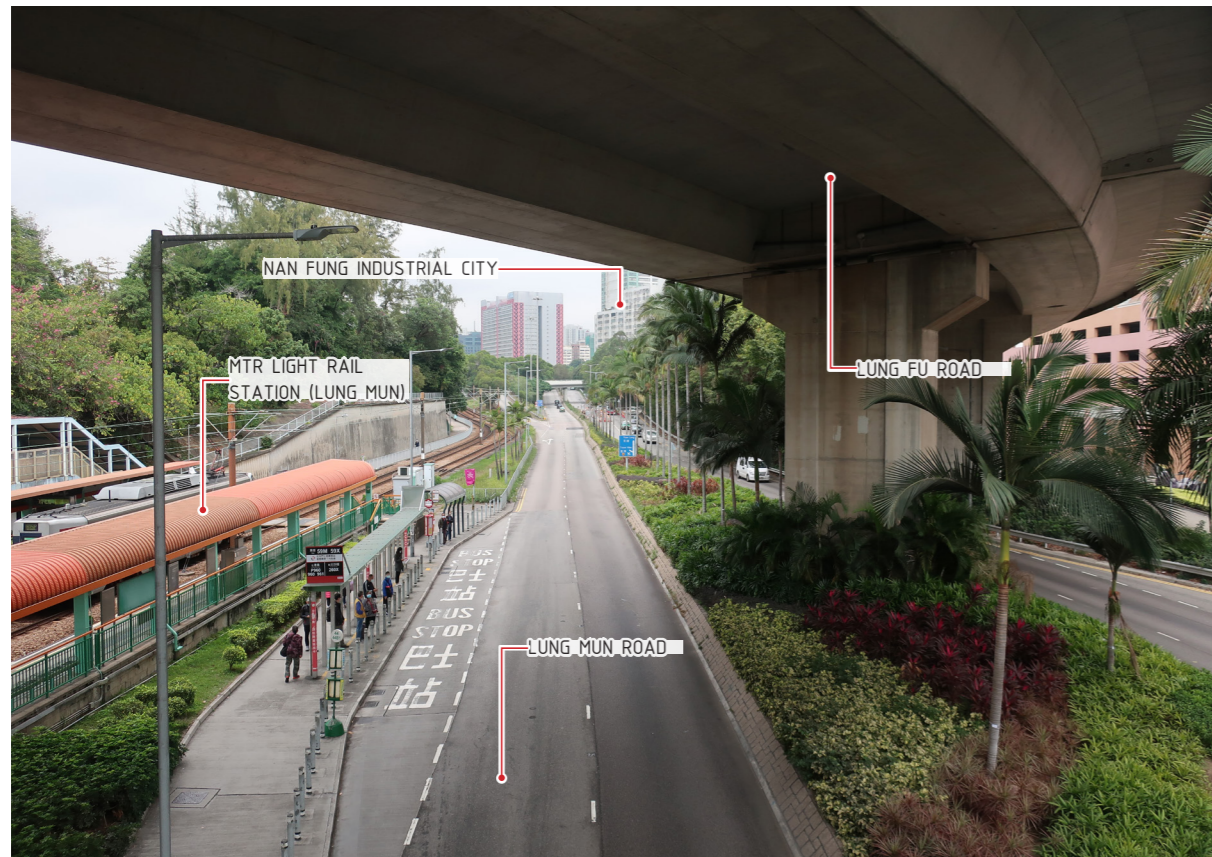
VP01 - FOOTBRIDGE ON LUNG MUN ROAD - EXISTING SITE CONDITION
