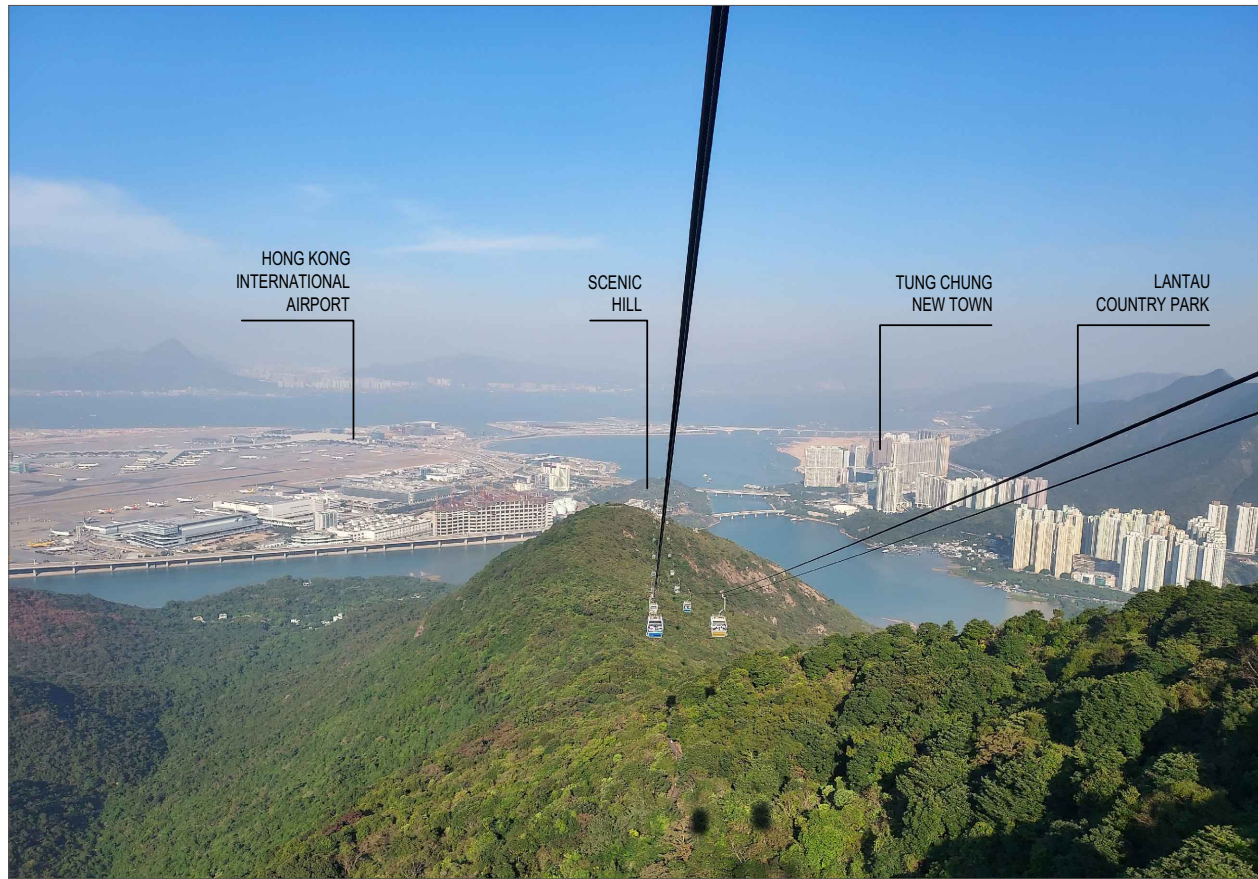
VP5 (from Cable Car of Ngong Ping 360): Existing Condition
