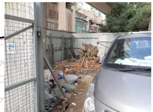
PHOTO 4947: TEMPORARY STORAGE AREA FOR CONSTRUCTION WASTE (DATE TAKEN: 22 DECEMBER 2021)
