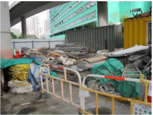
PHOTO 9669: CONSTRUCTION MATERIAL STORAGE (DATE TAKEN: 22 DECEMBER 2021)
