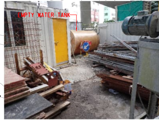
PHOTO 4961: SITE OFFICE (DATE TAKEN: 22 DECEMBER 2021)
