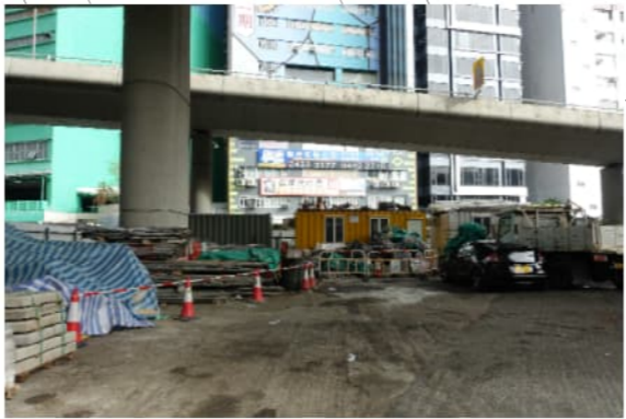
PHOTO 8857: CONSTRUCTION MATERIAL STORAGE AND SITE OFFICES (DATE TAKEN: 22 DECEMBER 2021)
