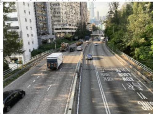
PHOTO 1119: TSUEN WAN ROAD (DATE TAKEN: 16 NOVEMBER 2021)
