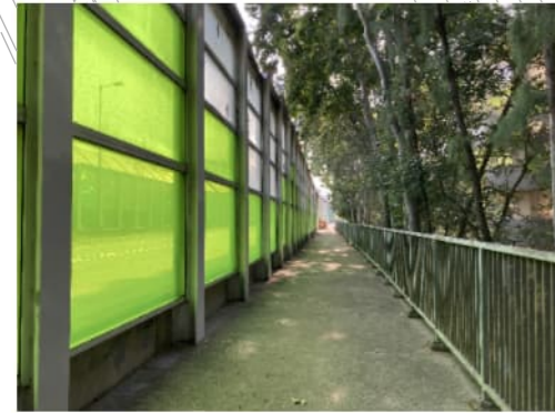
PHOTO 1103: NOISE BARRIER OF TSING TSUEN ROAD (DATE TAKEN: 16 NOVEMBER 2021)
