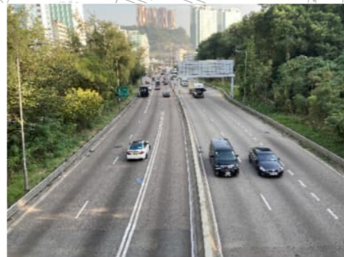
PHOTO 1120: TSUEN WAN ROAD (DATE TAKEN: 16 NOVEMBER 2021)
