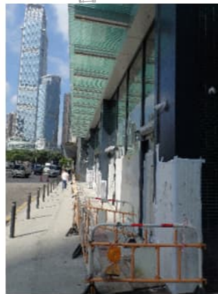
PHOTO 4527: FOOTPATH OUTSIDE 250-254 TEXACO ROAD (DATE TAKEN: 16 NOVEMBER 2021)
