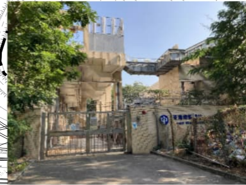
PHOTO 1084: TSUEN WAN SOUTH SUBSTATION (DATE TAKEN: 16 NOVEMBER 2021)
