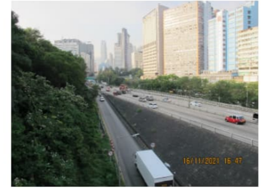
PHOTO 9148: TSUEN WAN ROAD AND SLOPE OF KWAI CHUNG PARK (DATE TAKEN: 16 NOVEMBER 2021)
