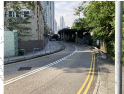
PHOTO 1083: WING TAK STREET (DATE TAKEN: 16 NOVEMBER 2021)
