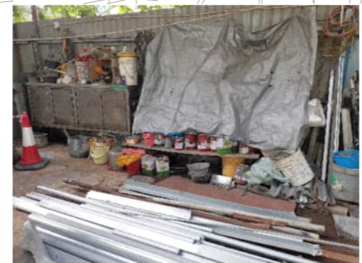
PHOTO 4969: CHEMICAL STORAGE AREA (DATE TAKEN: 22 DECEMBER 2021)
