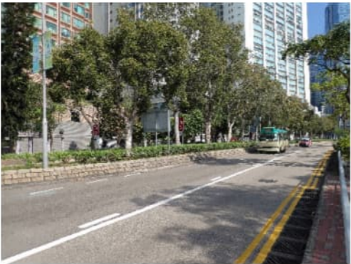
PHOTO 4408: HOI ON ROAD (DATE TAKEN: 16 NOVEMBER 2021)
