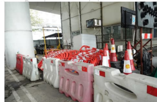
PHOTO 9025: MATERIAL STORAGE AREA (DATE TAKEN: 22 DECEMBER 2021)
