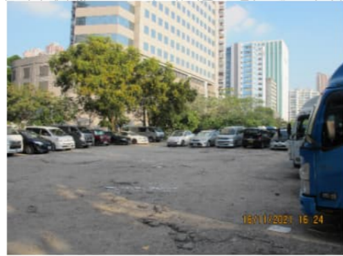
PHOTO 9100: OPEN CAR PARK (STT3750K&T) (DATE TAKEN: 16 NOVEMBER 2021)
