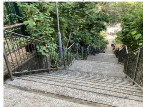
PHOTO 1123: STAIRS AND VEGETATION (DATE TAKEN: 16 NOVEMBER 2021)
