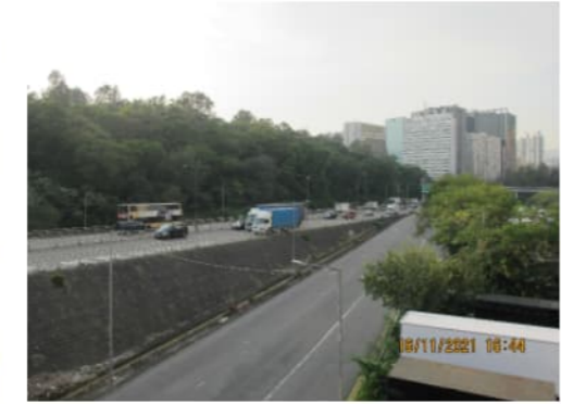
PHOTO 9133: TSUEN WAN ROAD (DATE TAKEN: 16 NOVEMBER 2021)
