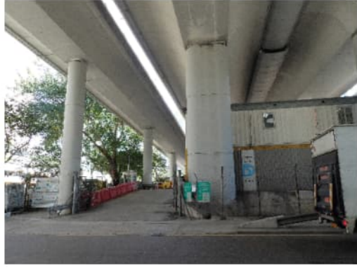
PHOTO 4435: HOI KOK STREET AND DSD MAINTENANCE DEPOT (DATE TAKEN: 16 NOVEMBER 2021)
