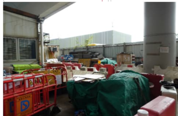
PHOTO 9029: MATERIAL STORAGE AREA (DATE TAKEN: 22 DECEMBER 2021)
