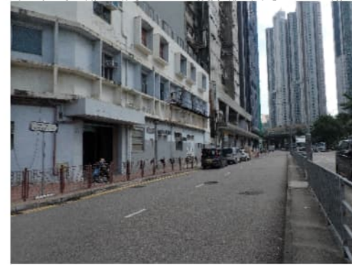
PHOTO 4516: TEXACO ROAD (DATE TAKEN: 16 NOVEMBER 2021)
