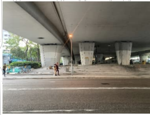
PHOTO 1179: LAMP POST NO. FC1383 AND CONTAINER PORT ROAD (DATE TAKEN: 16 NOVEMBER 2021)
