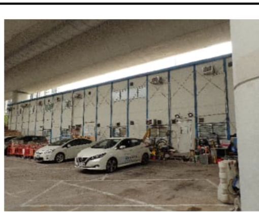
PHOTO 5016: DSD SITE OFFICE (DATE TAKEN: 22 DECEMBER 2021)
