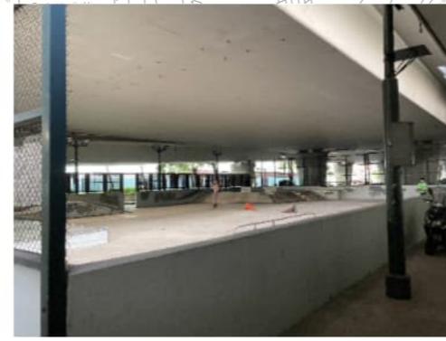
PHOTO 1165: KWAI SHUN STREET PLAYGROUND (DATE TAKEN: 16 NOVEMBER 2021)
