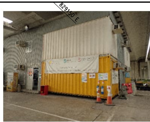
PHOTO 5001: CONTRACTOR SITE OFFICE (DATE TAKEN: 22 DECEMBER 2021)
