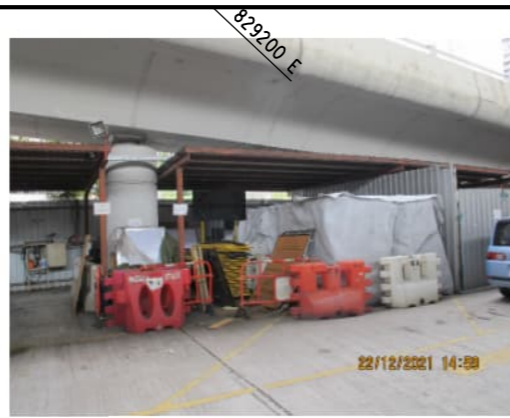
PHOTO 9767: MATERIAL STORAGE AREA (DATE TAKEN: 22 DECEMBER 2021)
