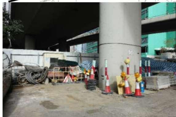
PHOTO 8851: CONSTRUCTION MATERIAL STORAGE IN OPEN AREA (DATE TAKEN: 22 DECEMBER 2021)
