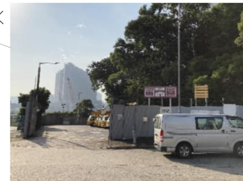
PHOTO 1091: WORKS SITE OF CONTRACT NO. 03/HY/2019 AND SLOPE (DATE TAKEN: 16 NOVEMBER 2021)
