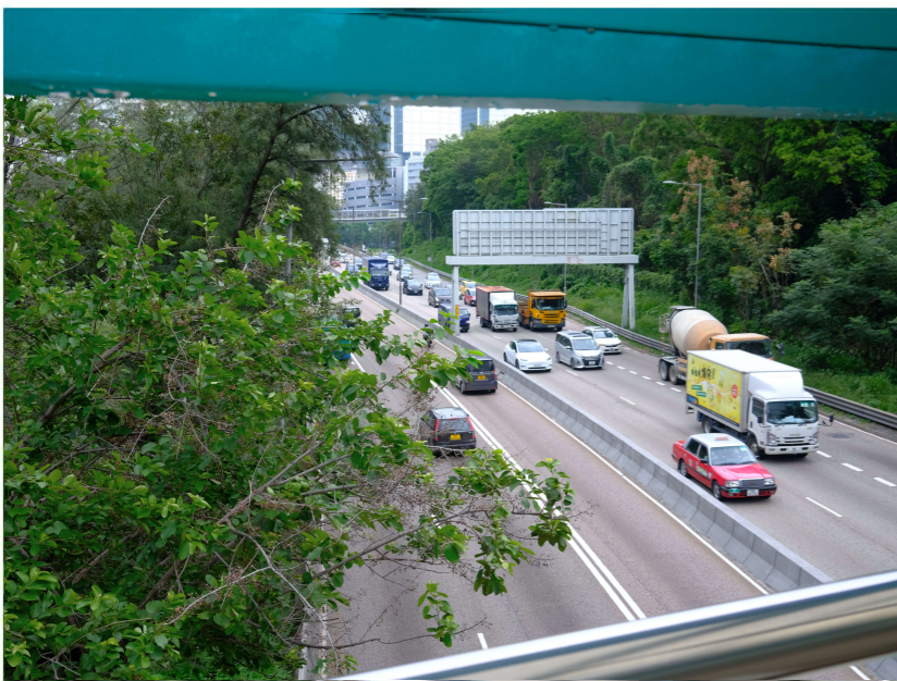
VPO7 FOOTBRIDGE TO KWAI CHUNG PARK
