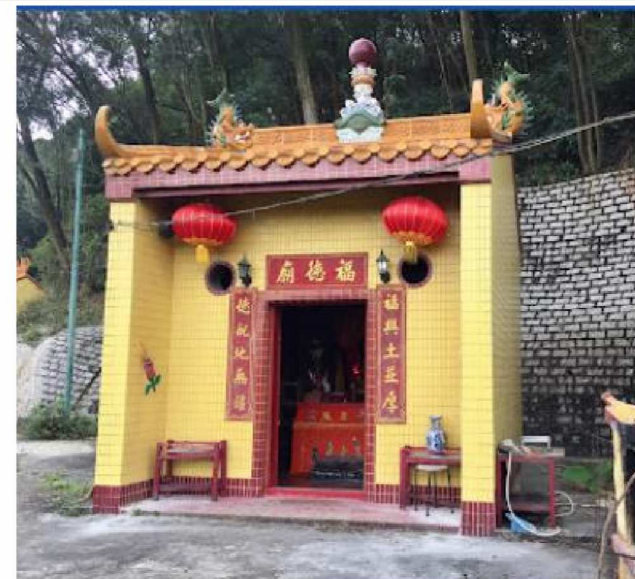
Fuk Tak Temple; looking southeast
