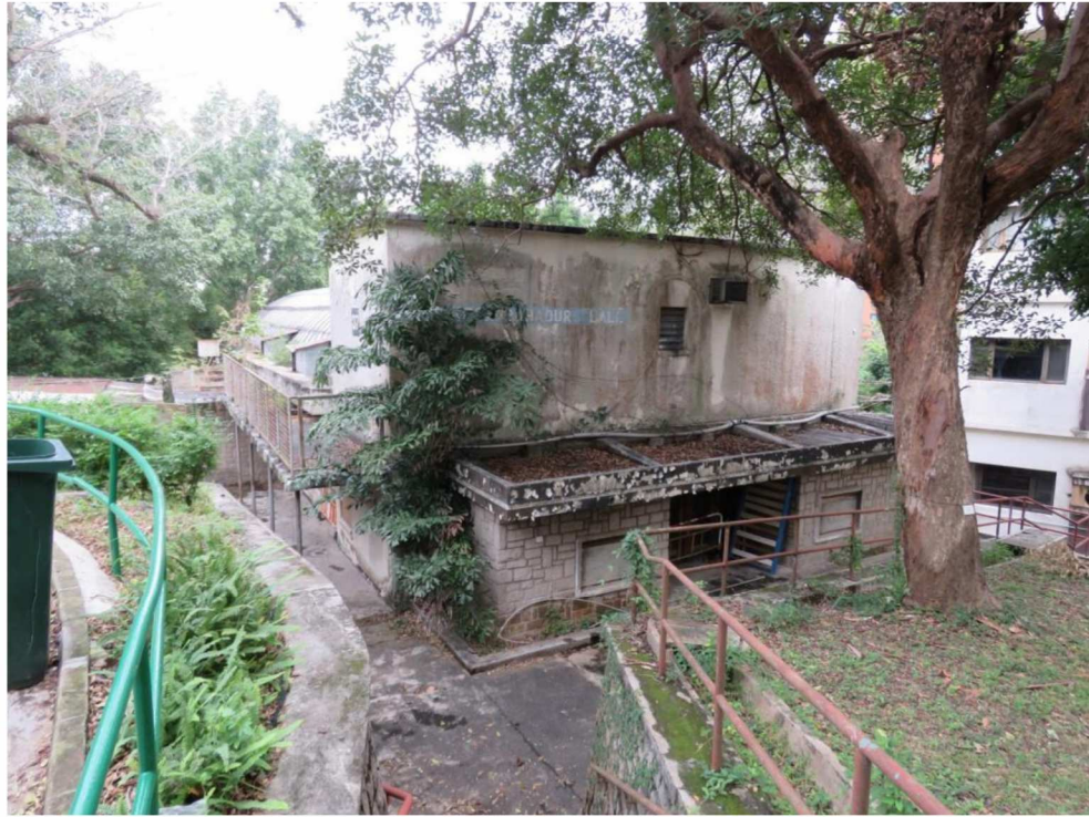
General view of GB-02, showing west and north facing elevations, looking southeast.
