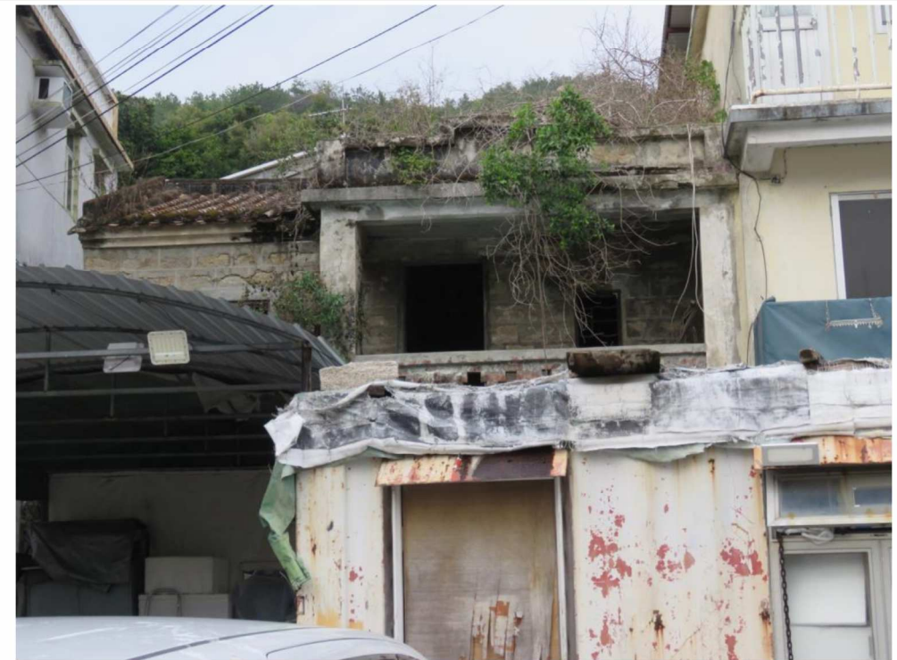
Close-in view of upper facade, looking north.
