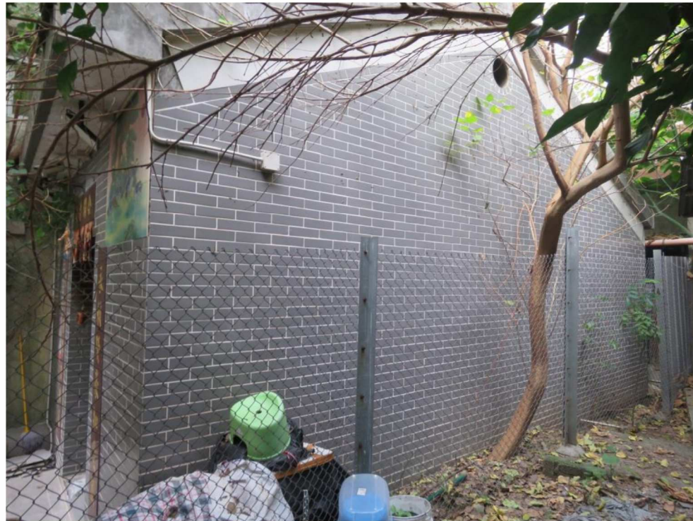
Side view of HB-29, showing east facing elevation, looking northwest.
