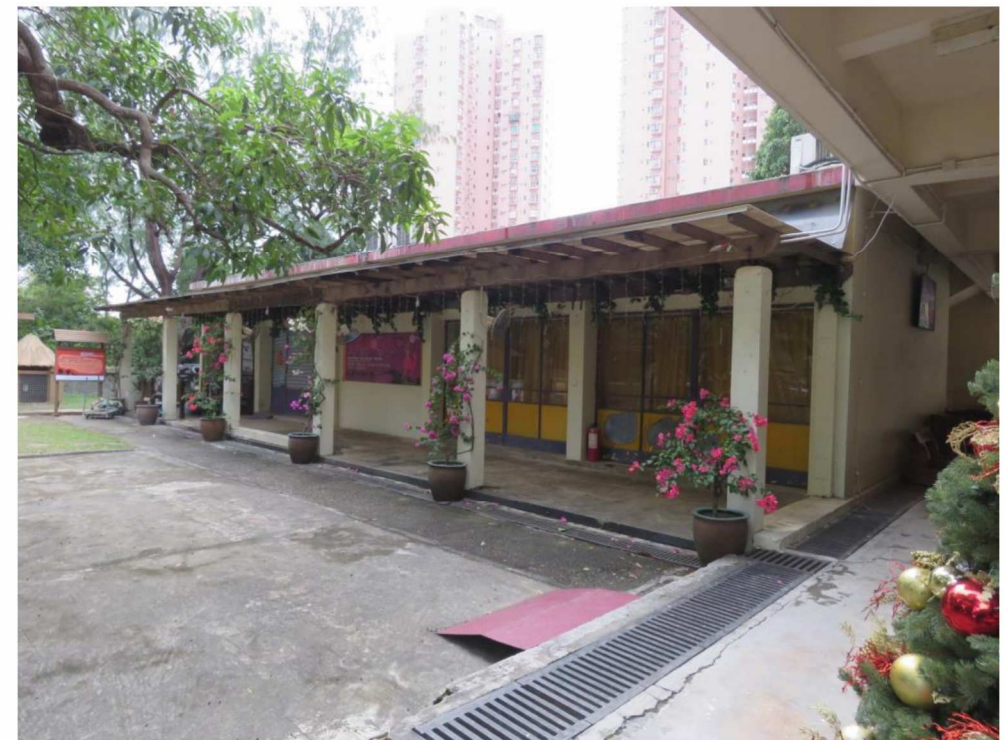
Side view, showing northeast facing elevation, looking southeast.
