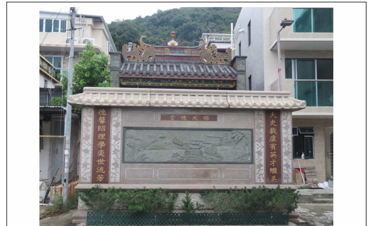
Front view of GB-07, showing modern style screen wall added in front, looking northeast.
