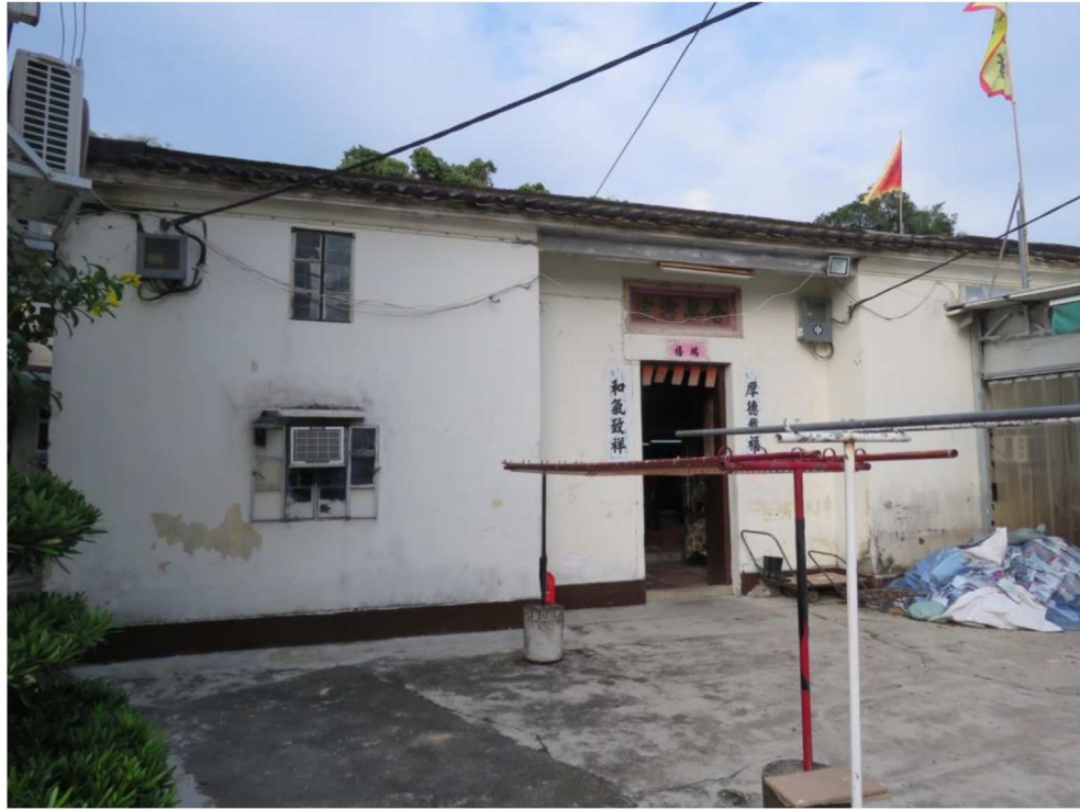
Façade view of GB-05, showing southwest facing elevation, looking northeast.
