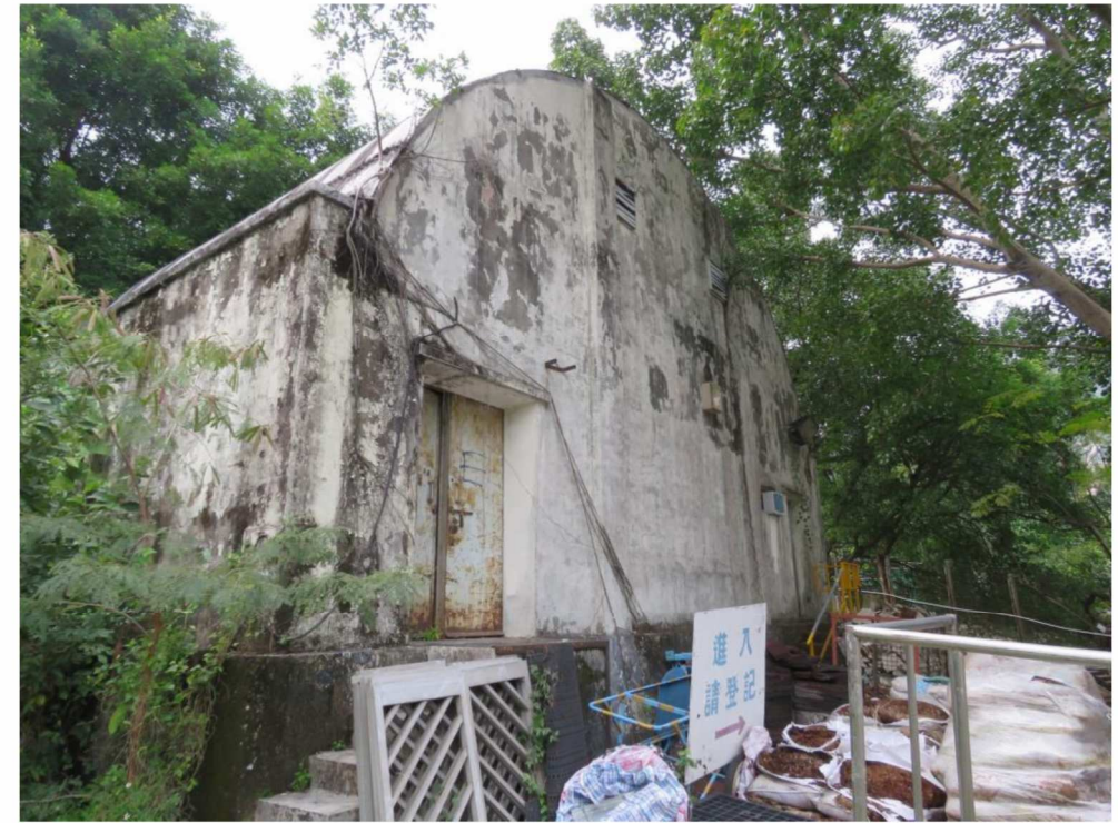
Rear view of GB-02, showing west facing elevation, looking northwest.
