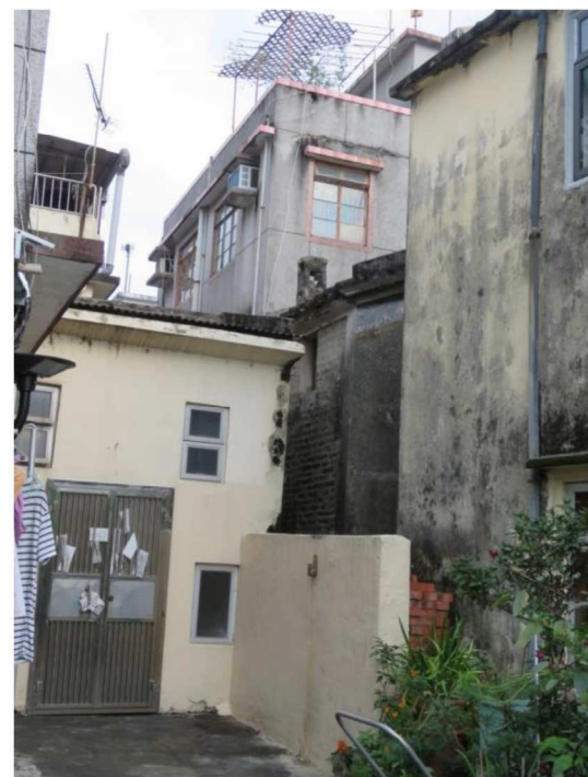
Entrance façade of HB-22, showing west-southwest facing elevation, looking east.
