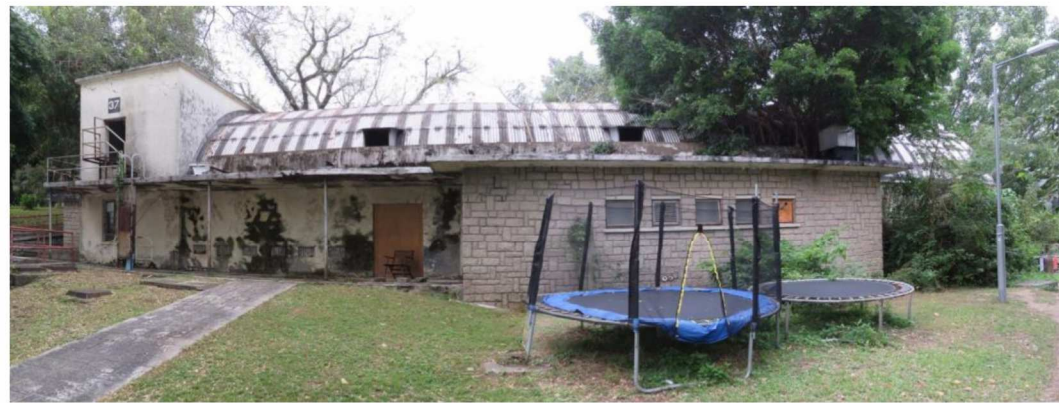
Panorama view of GB-02, showing south facing elevation, looking north.
