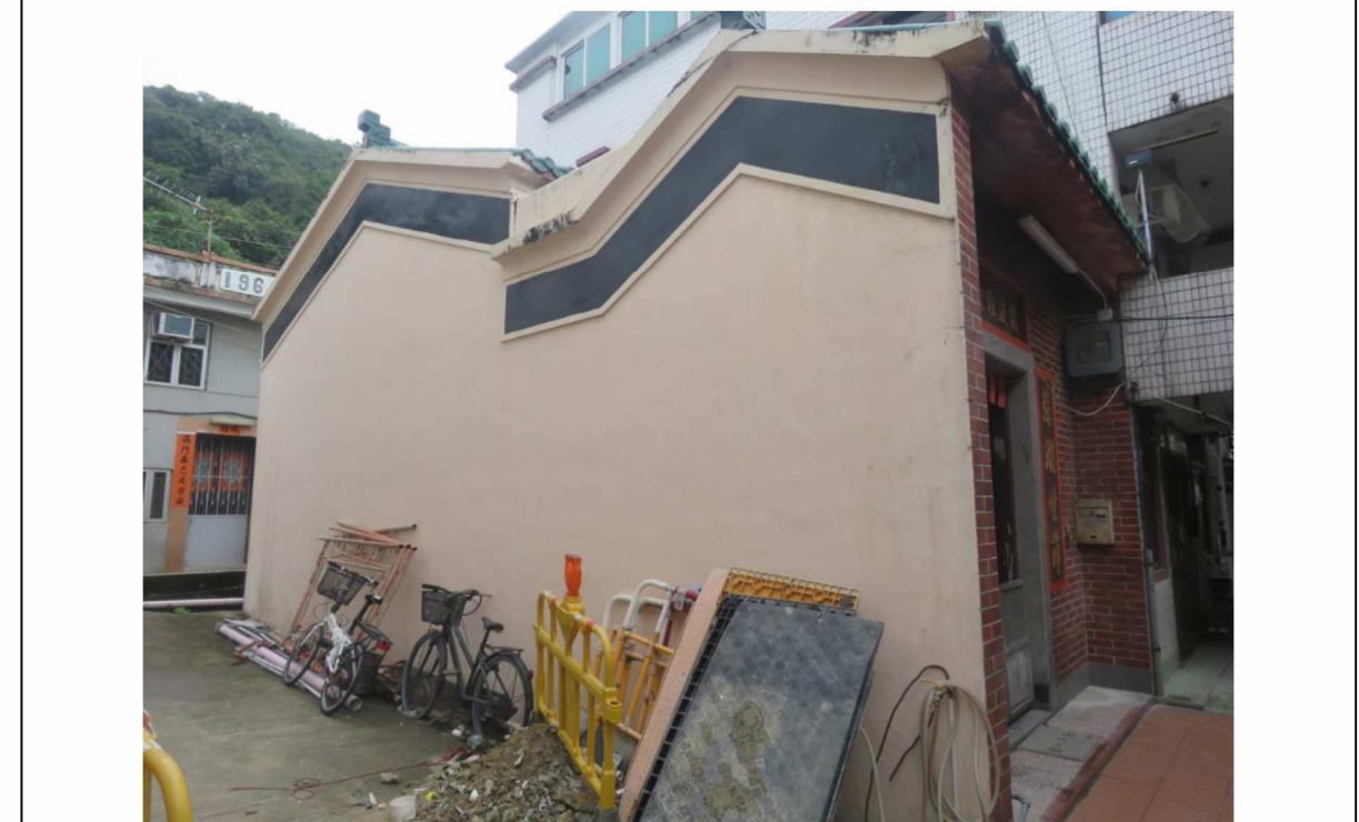
Front and side view of HB-02, showing southwest and northwest facing elevations, looking east.
