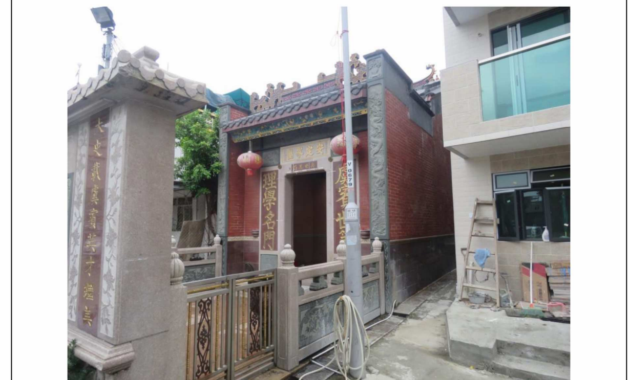
Façade view of GB-07, showing Modern rebuilt, looking north.
