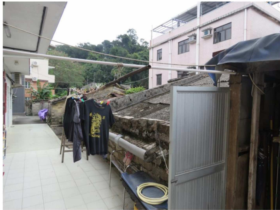
Rear view of HB-11, showing northeast facing elevation, looking east.
