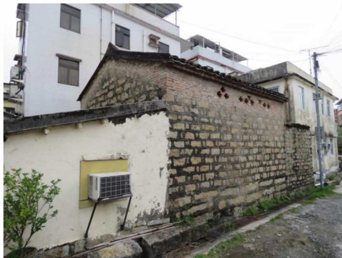
General view of HB-16, showing northwest and northeast elevations, looking south.
