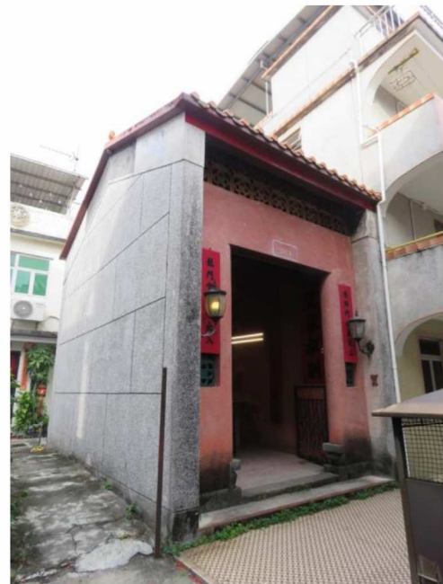
Façade view of HB-20, showing southeast facing elevation, looking northeast.
