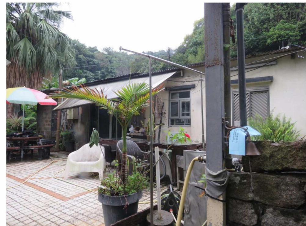
Close-in view of southern façade, looking southwest.
