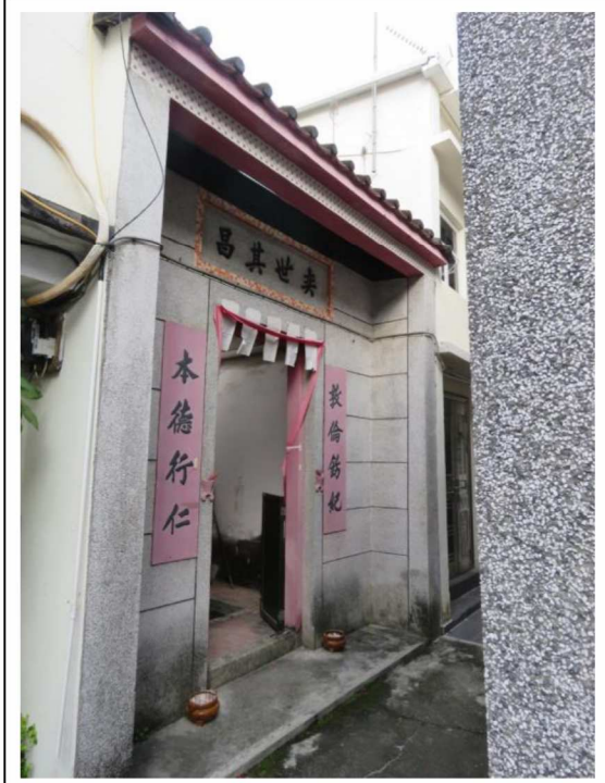
Façade view of HB-21, showing southeast facing elevation, looking northeast.
