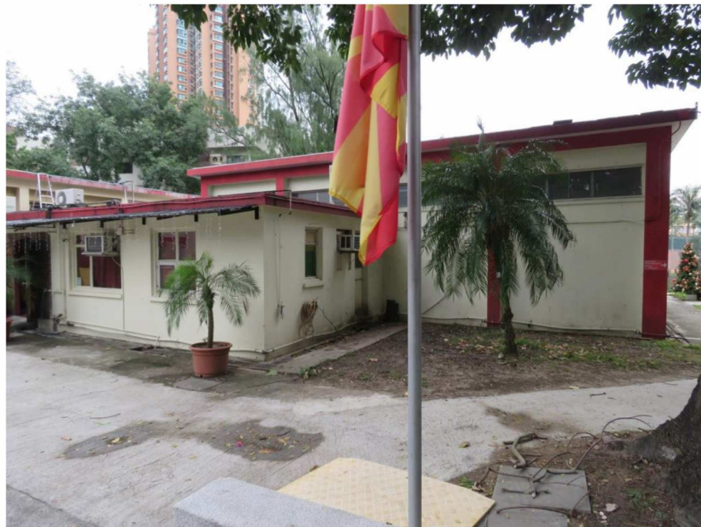
Front and side view of HB-27, showing entrance at northwest elevation and the building's northwest corners, looking southeast.
