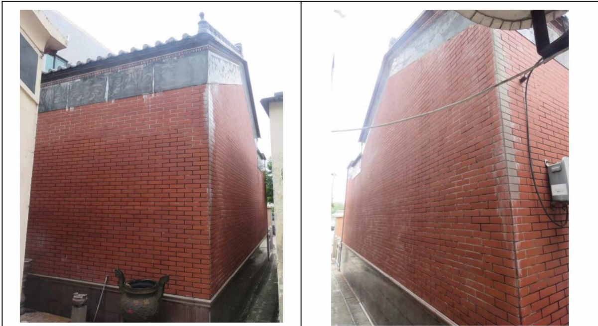
Rear and side view of GB-07, looking southwest.
