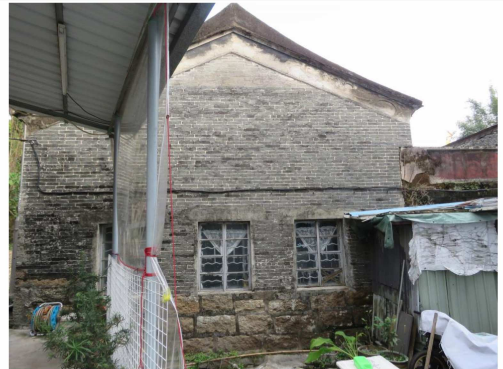
Rear part of southwest facing elevation, looking southeast.
