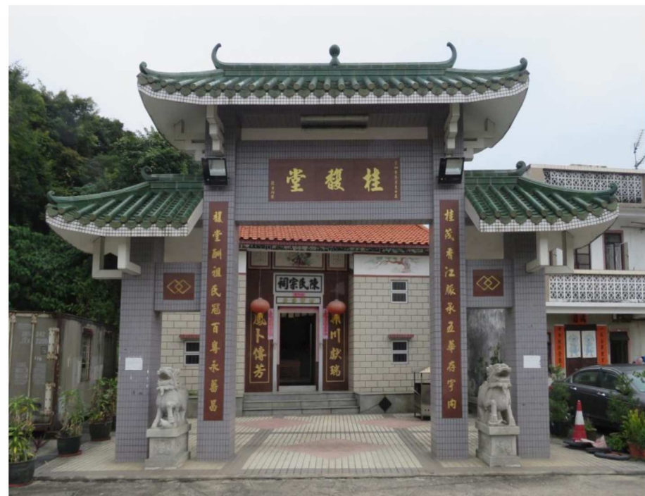
Entrance arch in front of GB-06, looking east-northeast.
