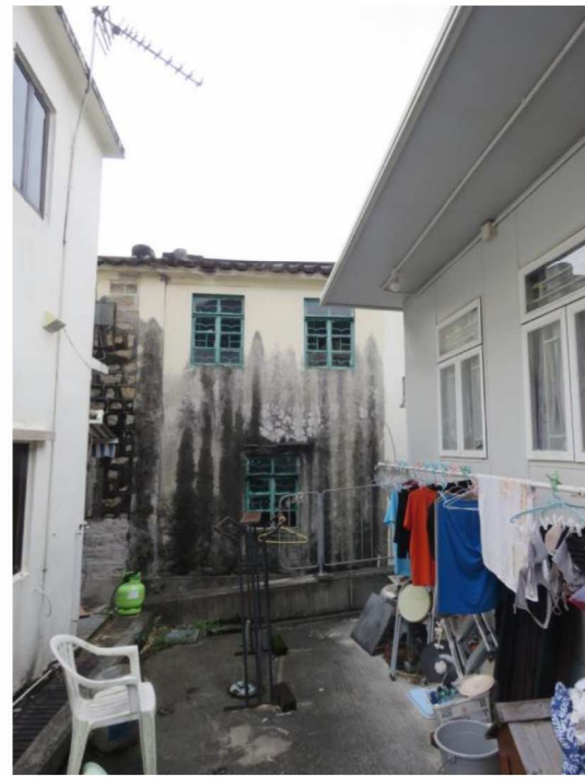
Rear view of No.8, showing northeast elevation, looking southwest.
