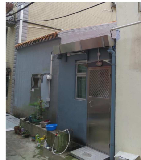
Rear view of HB-09, showing east-southeast facing elevation, looking southwest.
