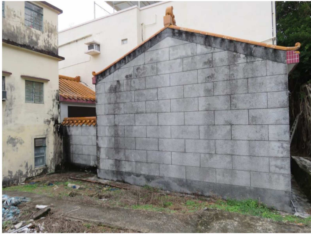
Side view of HB-14, showing southeast facing elevation, looking west.
