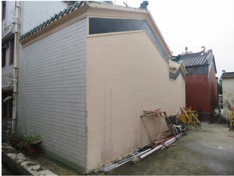
Rear and side view of HB-02, showing northeast and northwest elevations, looking south.
