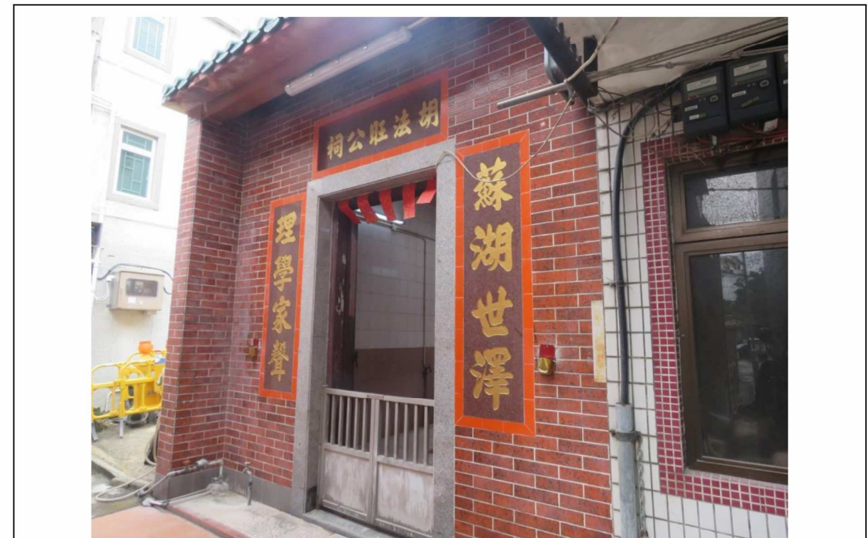
Façade view of HB-02, showing southwest facing elevation, looking north.
