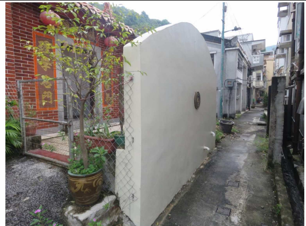
Screen wall in front of façade, looking east.
