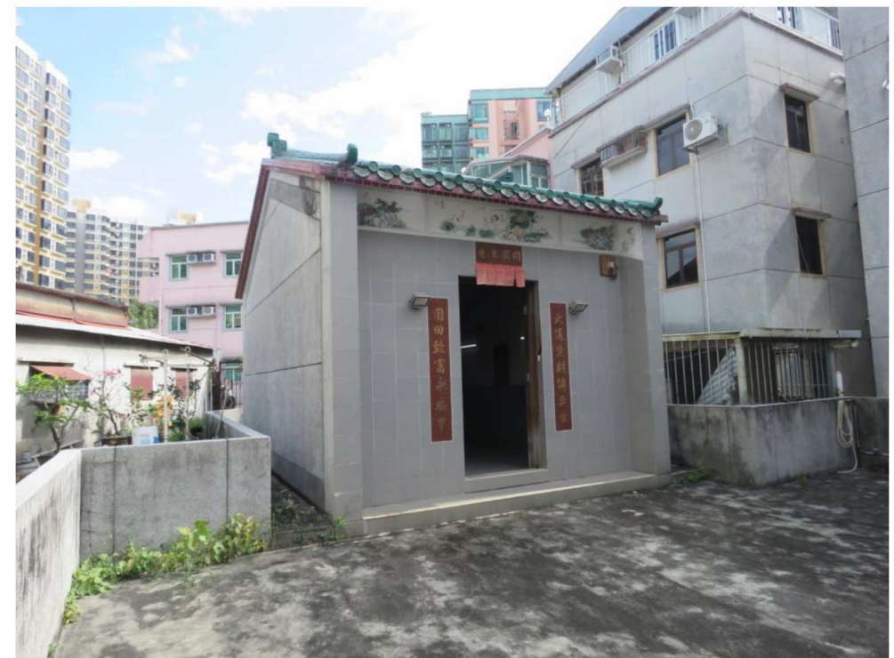
General view of HB-30, showing southwest and northwest facing elevations, looking east.
