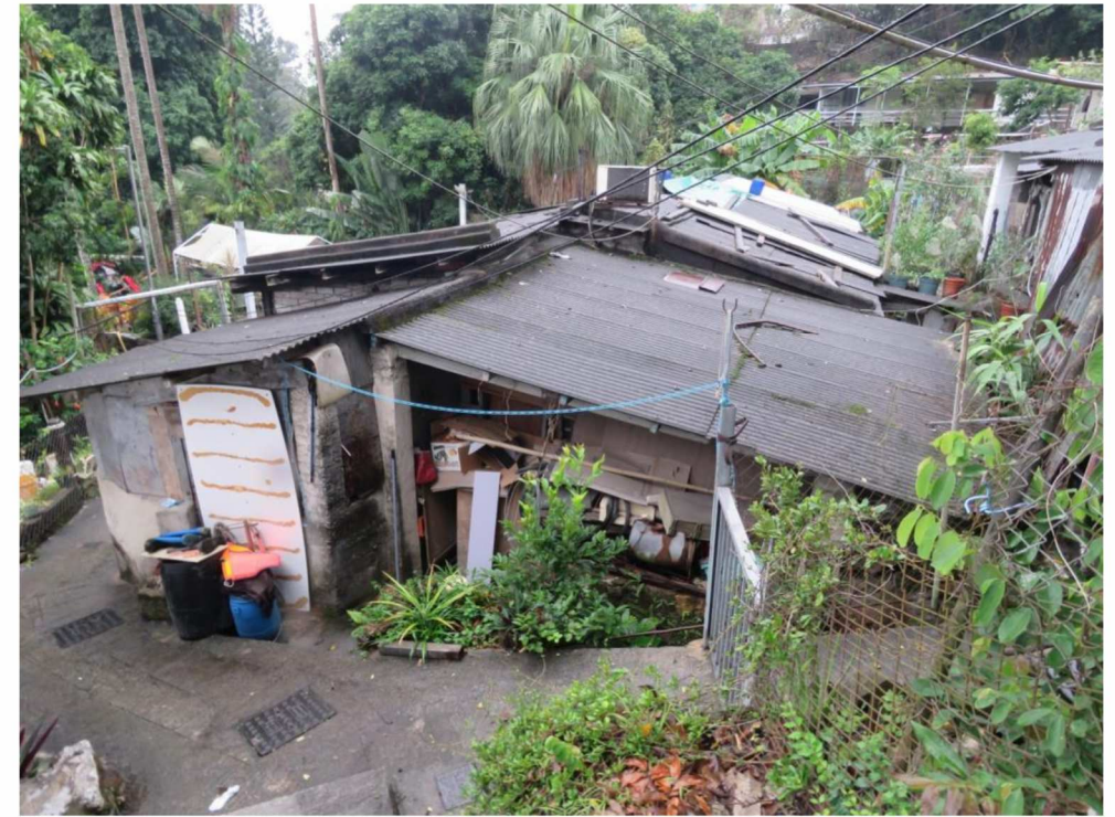
Side view of HB-01, showing northeast elevation, looking southwest.
