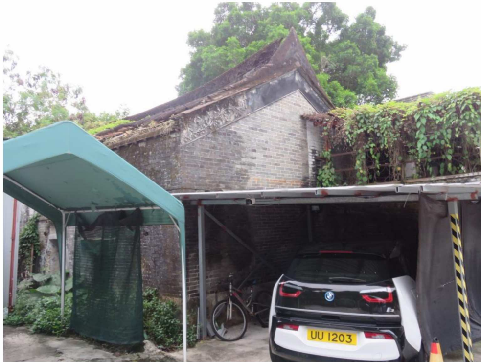
Looking southeast at northwest corner.
