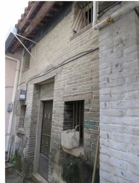
Façade view of No.84, showing southwest facing elevation, looking northwest.
