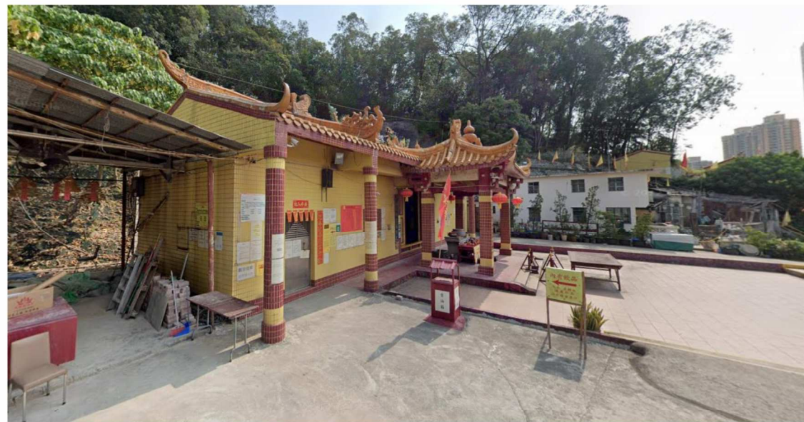
View of Nam On Buddhist Monastery main building; looking southwest
