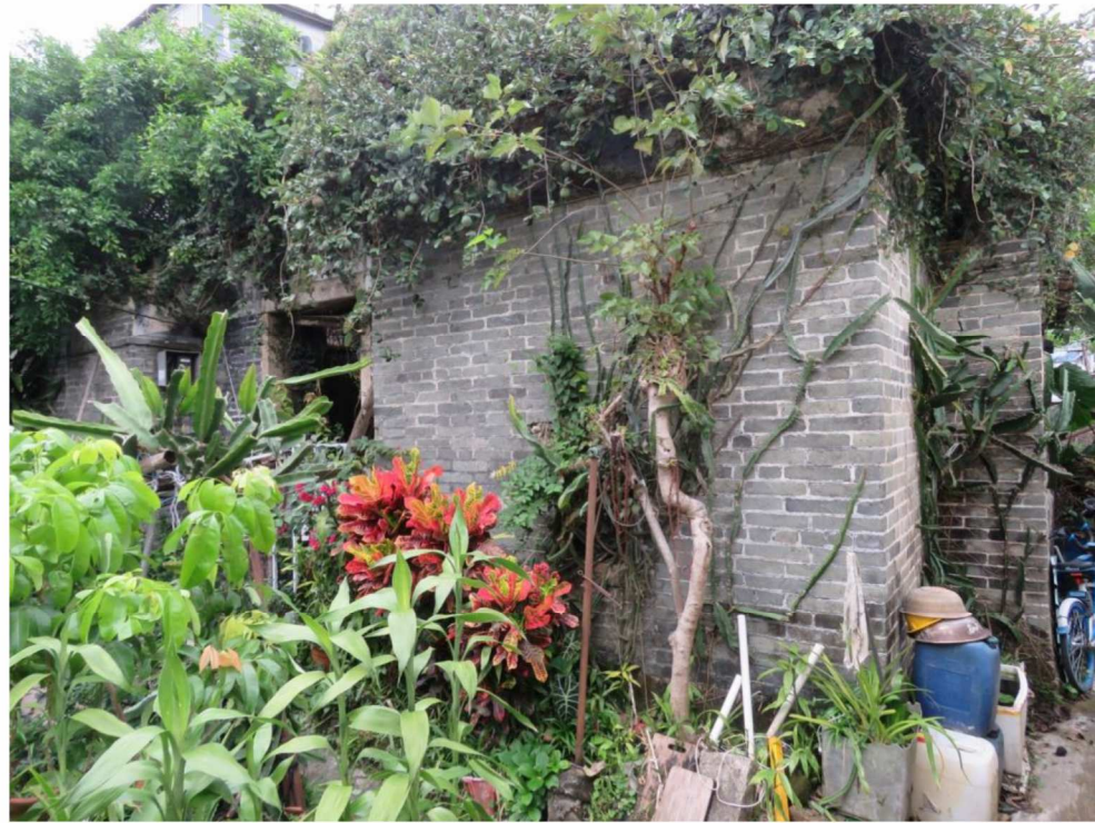
Façade and southeast corner of GB-05, looking north.
