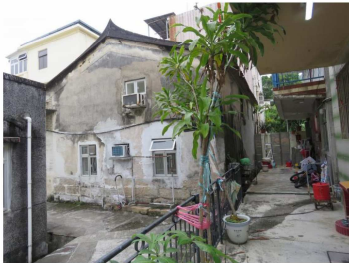
Side and rear view of HB-12, showing southeast and northeast elevations, looking west.
