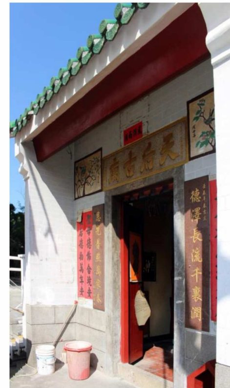
Façade view of HB-28, showing southeast facing elevation, looking northwest.
