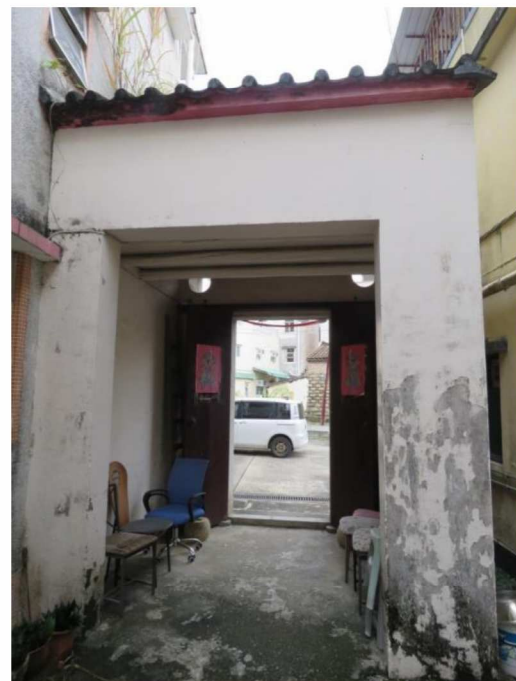
Rear view of HB-17, showing west facing elevation, looking east.
