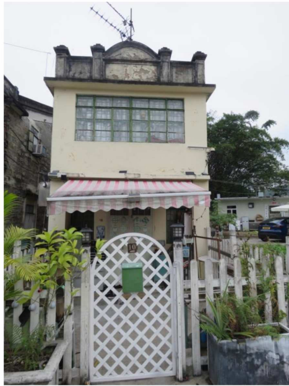
Façade view of HB-07, showing southwest facing elevation, looking northeast.
