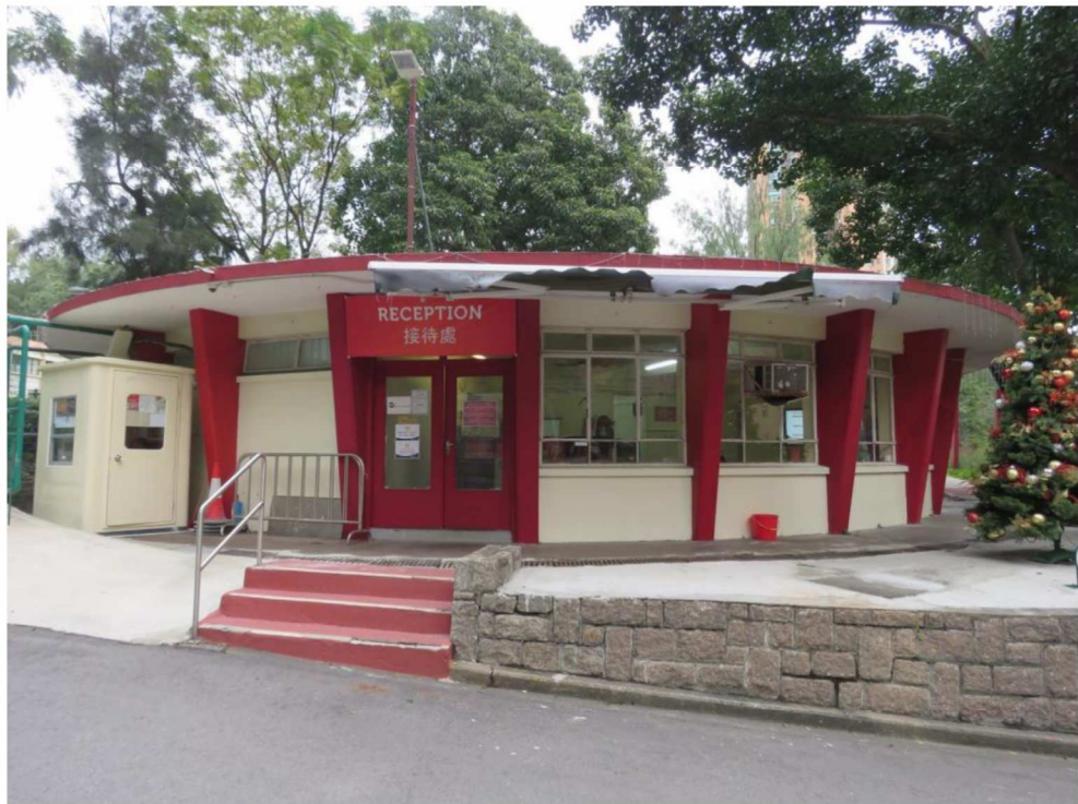
Front view of HB-26, showing entrance and round wall, looking northeast.
