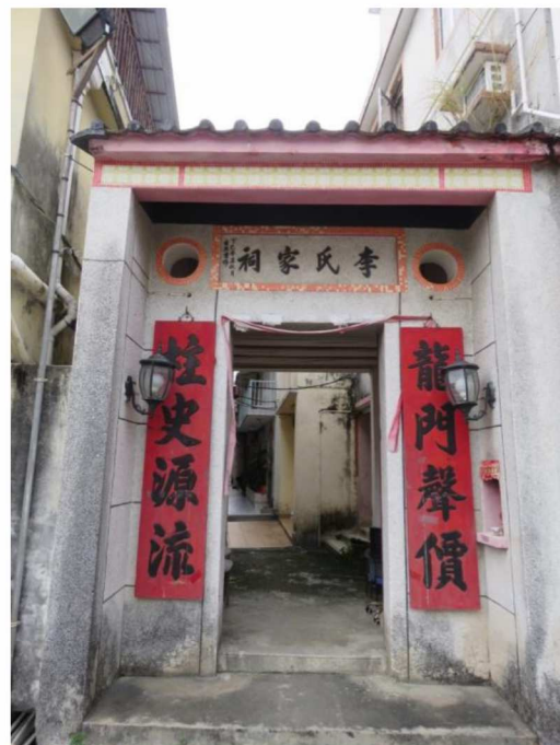
Façade view of HB-17, showing east facing elevation, looking west.
