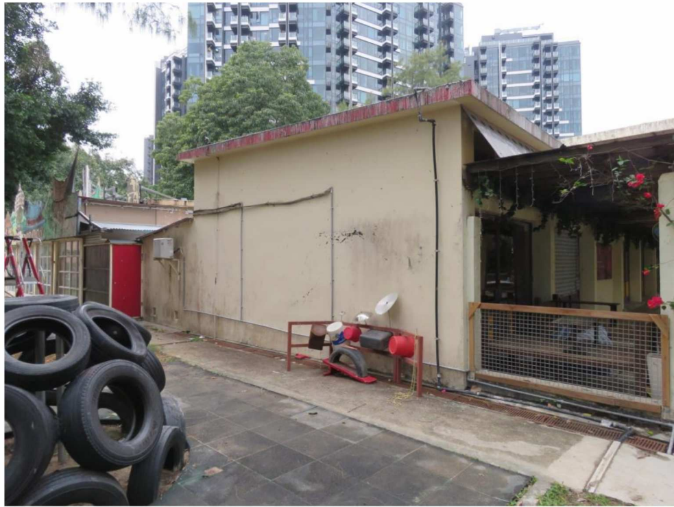
Rear view, showing southeast elevation, looking north.
