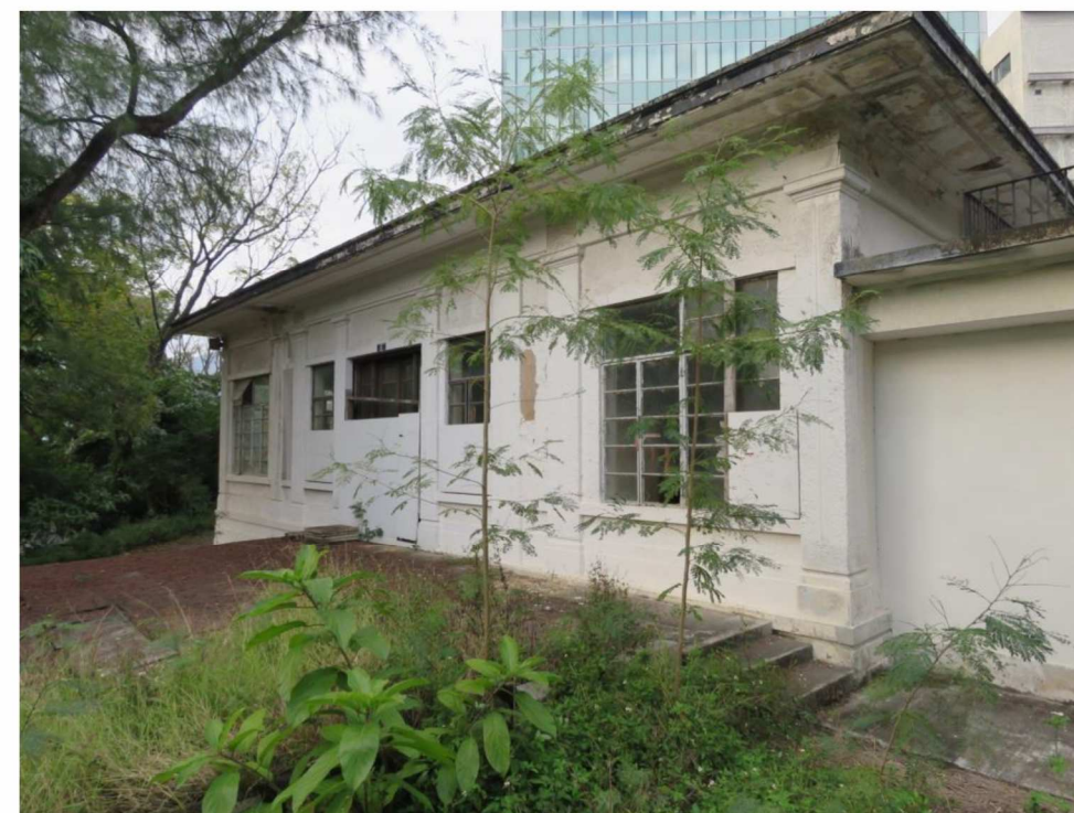
Rear view of GB-01, showing south facing elevation, looking northwest.
