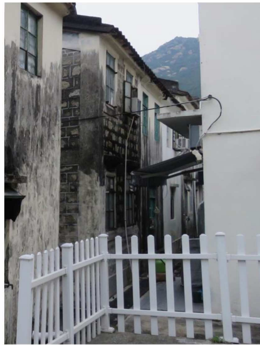
Rear view of HB-06, showing northeast elevation, looking northwest.
