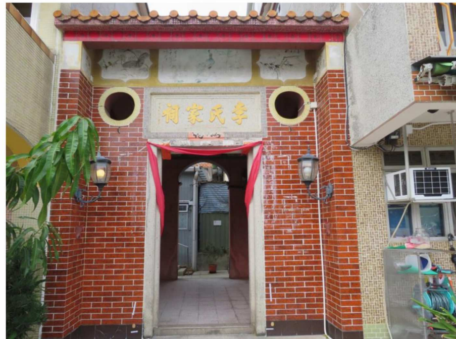
Façade view of HB-19, showing southeast facing elevation, looking northwest.
