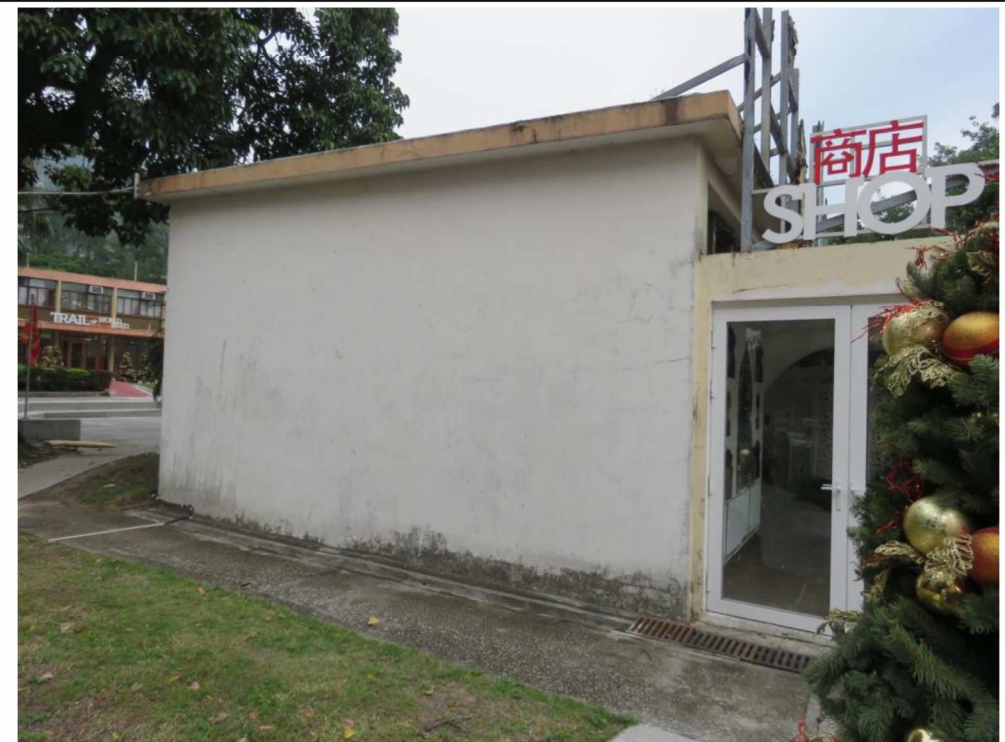
Side view, showing southwest facing elevation, looking east.
