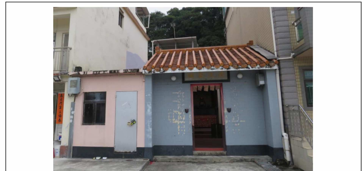
Façade view of HB-09, showing west-northwest facing elevation, looking east-southeast.
