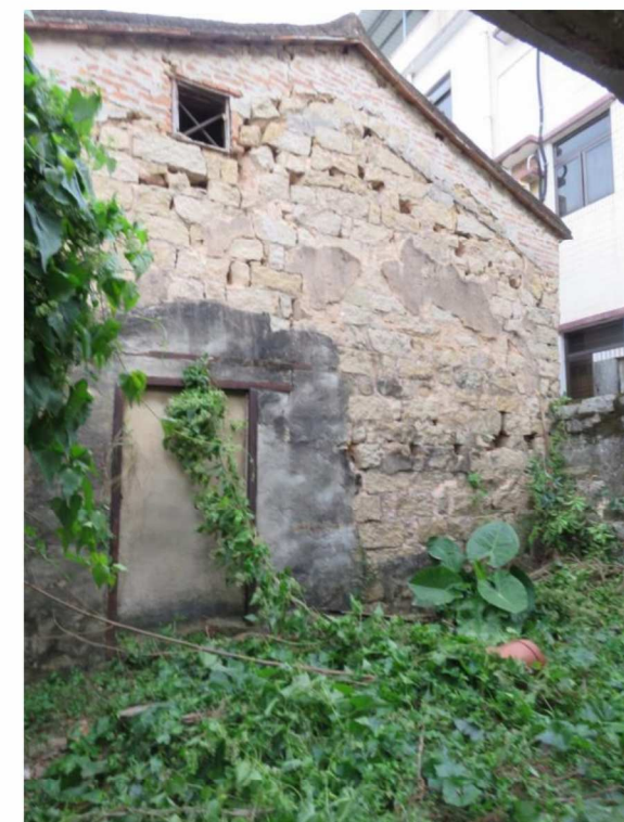
Sealed entrance on southeast elevation, looking northeast.
