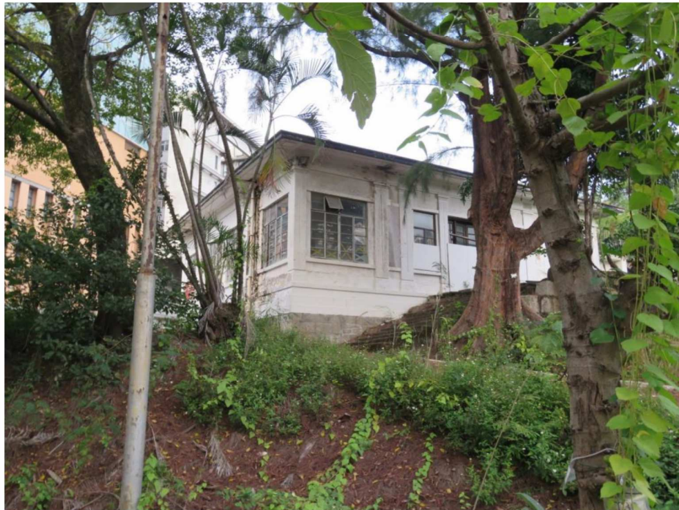
Looking northeast at southwest corner.
