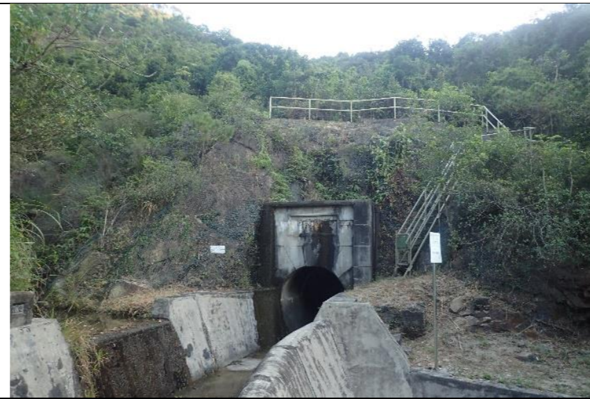
Southwestern entry of Tai Lam Chung Catchwater Tunnel No. 6
