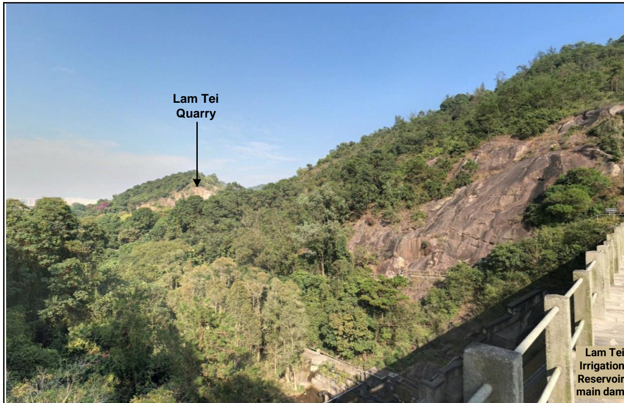
VP-LT10 – EXISTING CONDITION
