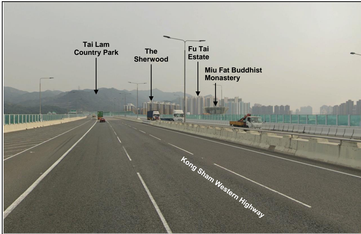
VP-LT7 – EXISTING CONDITION
