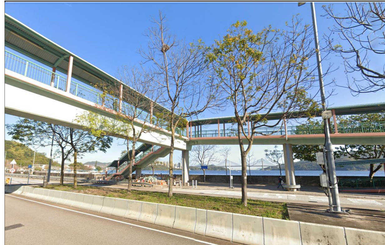
VSR-TL11 – Pedestrians on Footbridge across Castle Peak Road – Tsing Lung Tau
