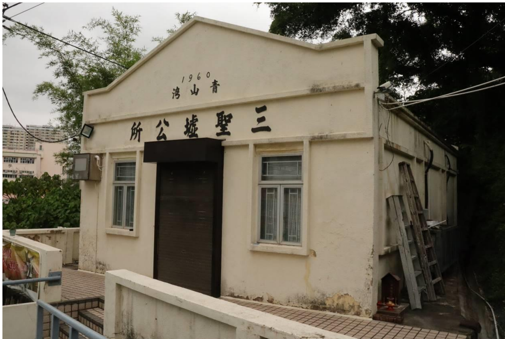
Southeast elevation of Castle Peak Sam Shing Hui Village Office
