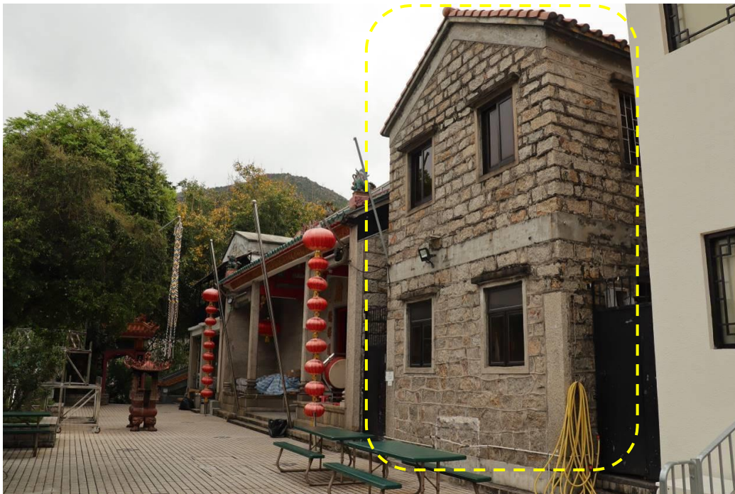
Southeast elevation of Tai Sui Din (Yellow dotted-line in the photo shows Tai Sui Din)
