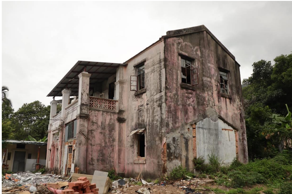
East elevation of Hung Lau
