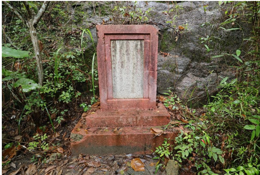
A memorial tablet next to the steps at the east end of the main dam of Lam Tei Reservoir
