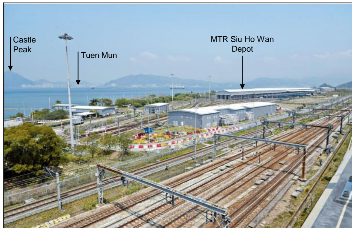
VSR-NL3 – Workers and Future Residents at MTR Siu Ho Wan Depot
