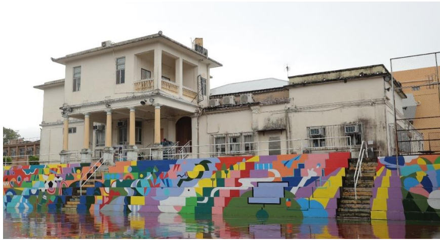
ELCHK Gloria Lutheran Church (View from Northeast to Southwest)
