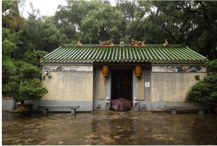
Southeast elevation of Sam Shing Temple (Fanling Wai)
