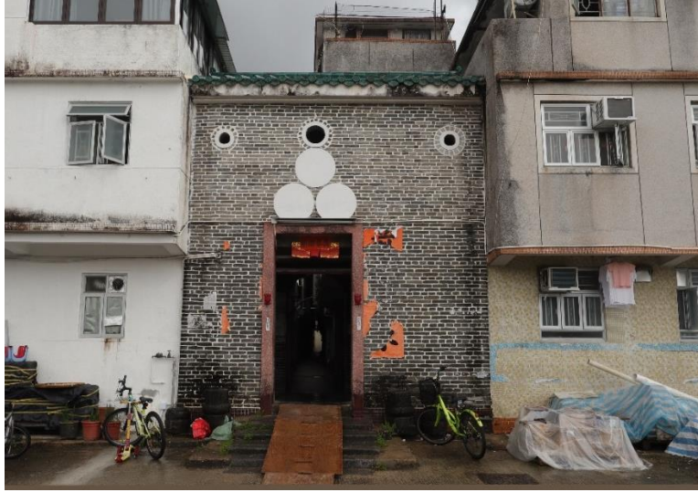
Front elevation of Fanling Wai, Entrance Tower
