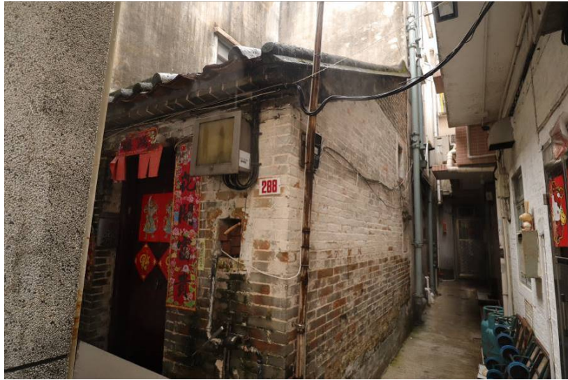
BH-04-25: No. 288 Village house, Orientation: Northwest
