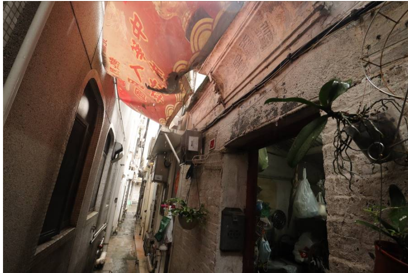
BH-04-18: No. 190 Village house, Orientation: Northwest
