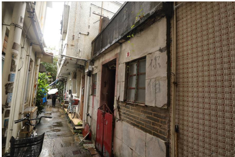
BH-04-8: No.30 Village house, Orientation: Northwest
