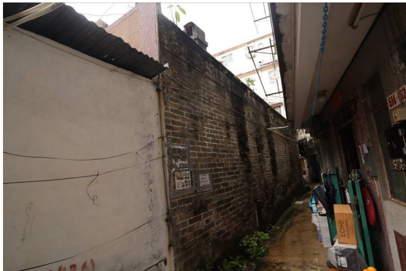
BH-04-30: No. 527 Village house, Orientation: Southwest, Rear View
