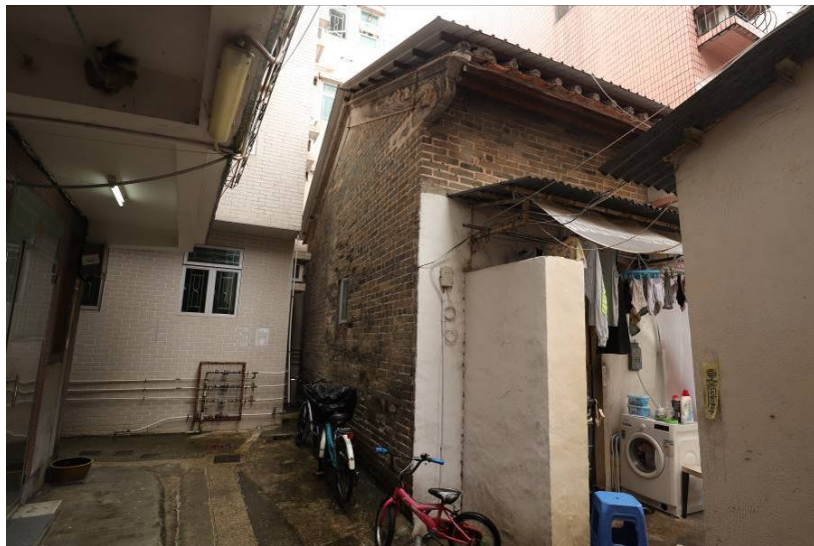
BH-04-29: No. 524-526 Village house, Orientation: Southwest
