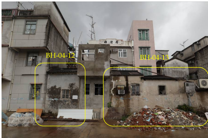
BH-04-12 and BH-04-13: No. 146 and 146B Village house, Orientation: Southeast, Rear view from northwest to southeast
