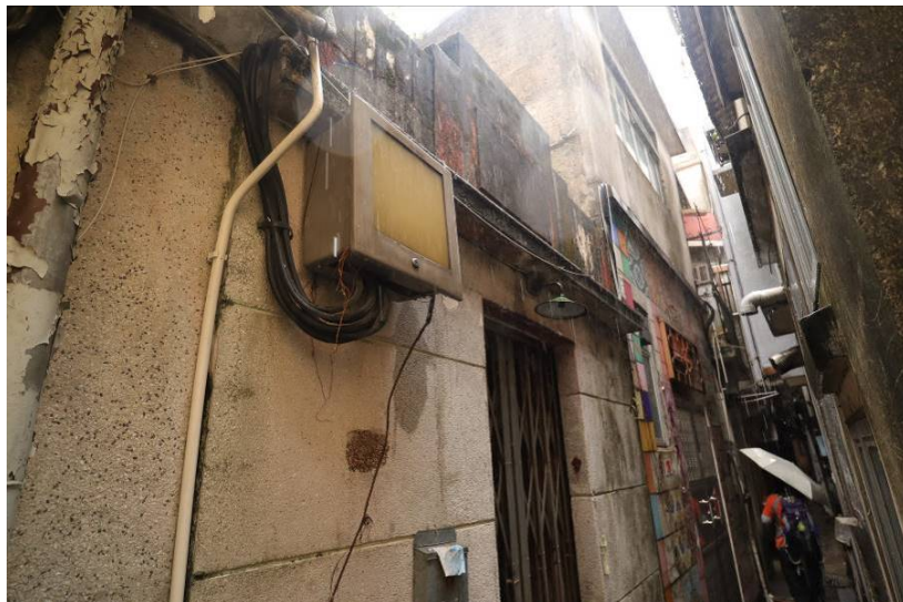
BH-04-24: No. 260 Village house, Orientation: Northwest
