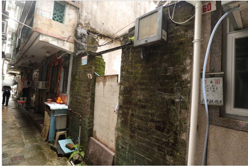
BH-04-10: No. 59 Village house (ruin), Orientation: Northwest
