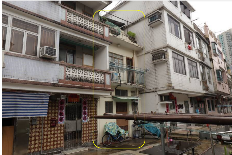
BH-04-28: No. 360 Village house, Orientation: Northwest
