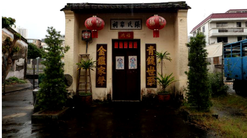
Front view of Cheung Ancestral Hall (Kai Leng)
