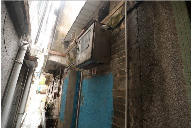
BH-04-7: No.19 Village house, Orientation: Northwest
