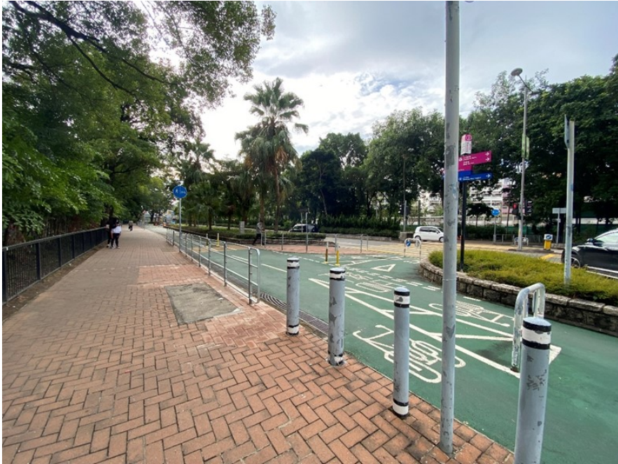
Photo 1: Pedestrian road and cycling track along San Wan Road
