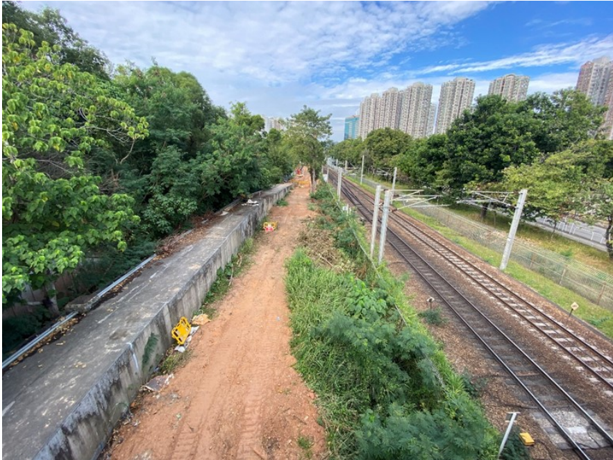
Photo 7: Top view from So Kwun Po Road (elevated road) to unpaved road along MTR railway
