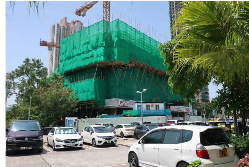
LR13.1 - CONSTRUCTION SITE
