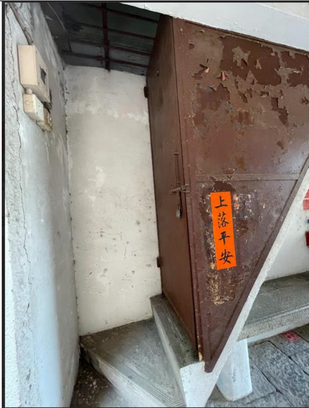
(Figure 23. View of the staircase)
