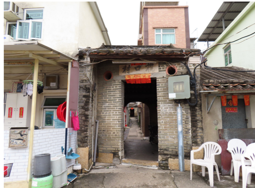
LR2.4 Entrance Gate, Lam Hau Tsuen 欖口村圍門
