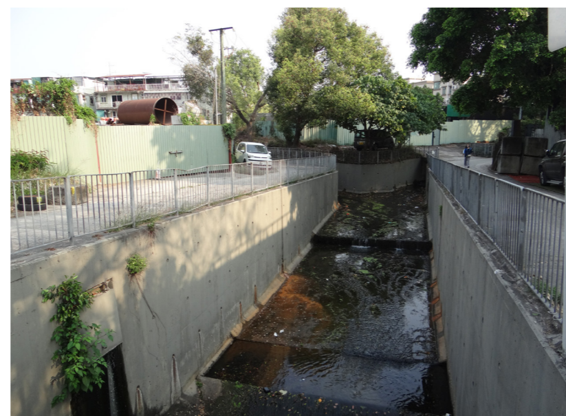
LR11 Channelized Watercourse
