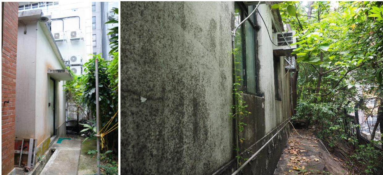
Figure 8.24. Extension of Red House in 2019.
