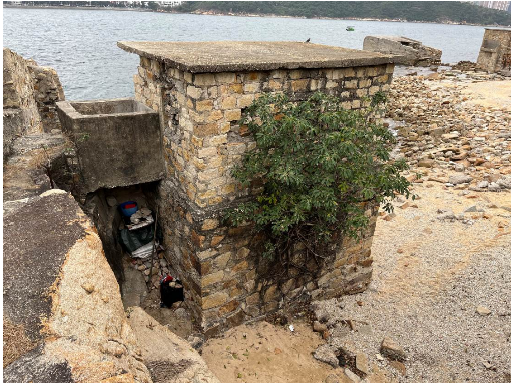
Plate 2.40. Northern elevation of the stone hut in the east of the site. A concrete well is attached to its side and connected to the seawall.
