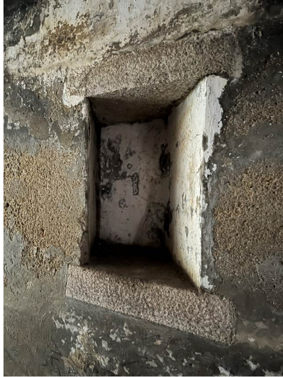
Plate 1.17. Recessed space on the wall for lamp placement. The lintel and base are formed by granite blocks.
