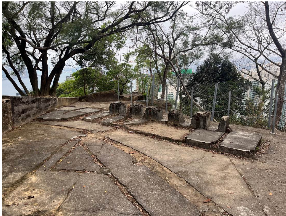
Plate 1.20. Remains of tracks and anchoring installations of Gough Battery.
