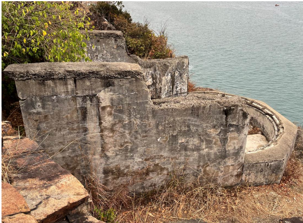
Plate 5.2. Side elevation of the northern coastal searchlight emplacement.
