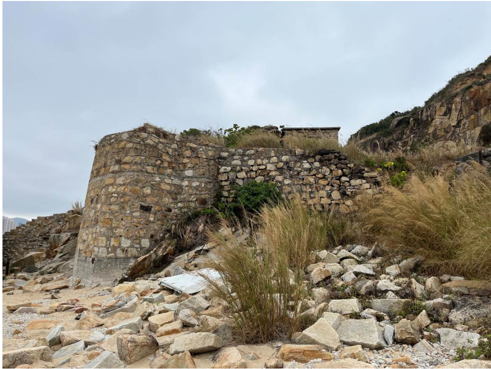
Plate 2.42. Curved stone wall behind the stone hut (checker's kiosk).
