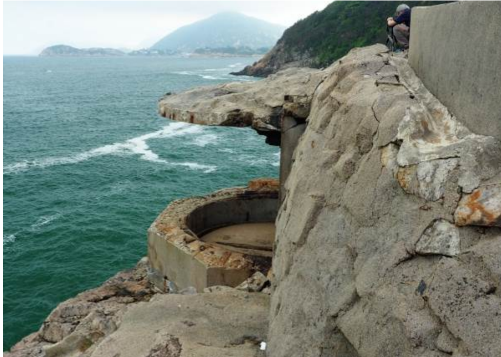
Plate 5.5. Photo of a searchlight emplacement at Cape Collinson Battery taken in 2018. A semi-circular roof can be observed in the photo.
