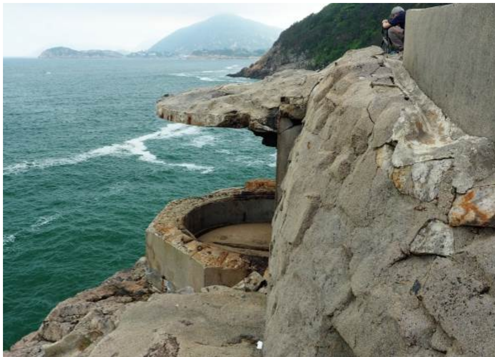
Plate 6.6. Photo of a searchlight emplacement at Cape Collinson Battery taken in 2018. A semi-circular roof can be observed in the photo.
