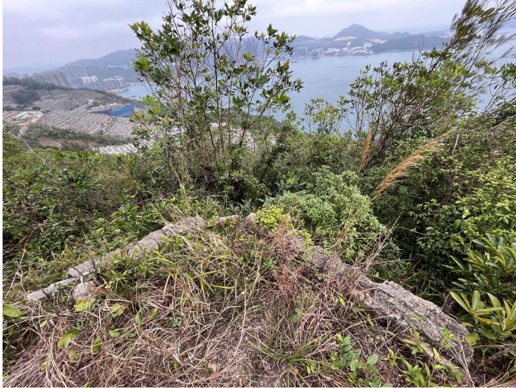
Plate 1.26. Remains of the caponier foundation.
