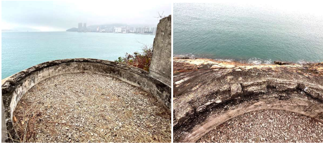
(Left) Plate 6.4. The front part of the southern coastal searchlight emplacement. A sliding track and gear teeth could be found along the inner profile.
