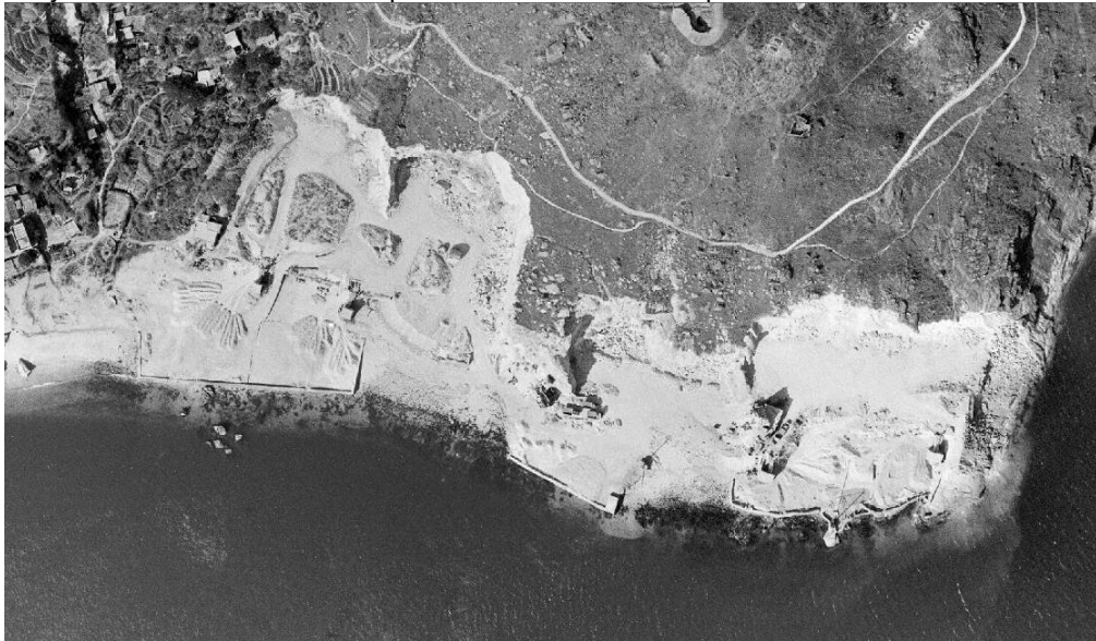
Plate 2.30. Quarries in Lei Yue Mun in 1963 34 . The extent of the quarries ranged from the end of the eastern end of the southern coast to the existing Ma Pui Village in the west.
