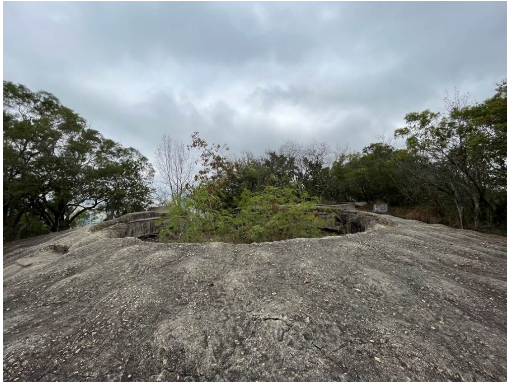
Plate 1.11. 9.2-inch gun emplacement of Gough Battery.
