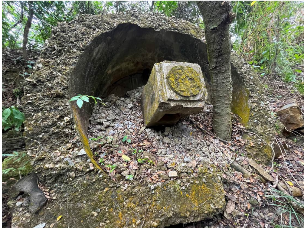
Plate 1.9. Collapsed depression range finder.
