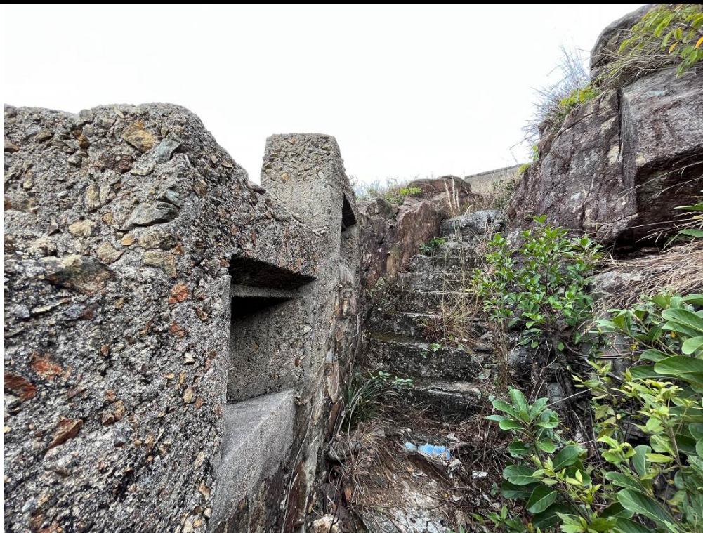
Plate 1.27. Firing trench with loopholes connecting the redoubt and the caponier.
