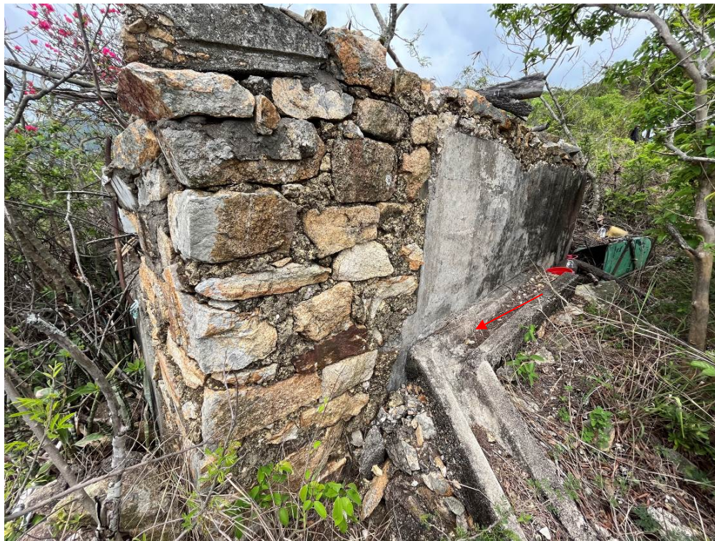
Plate 12.3. A drainage duct could be found attaching to the eastern façade (red arrow indicates).
