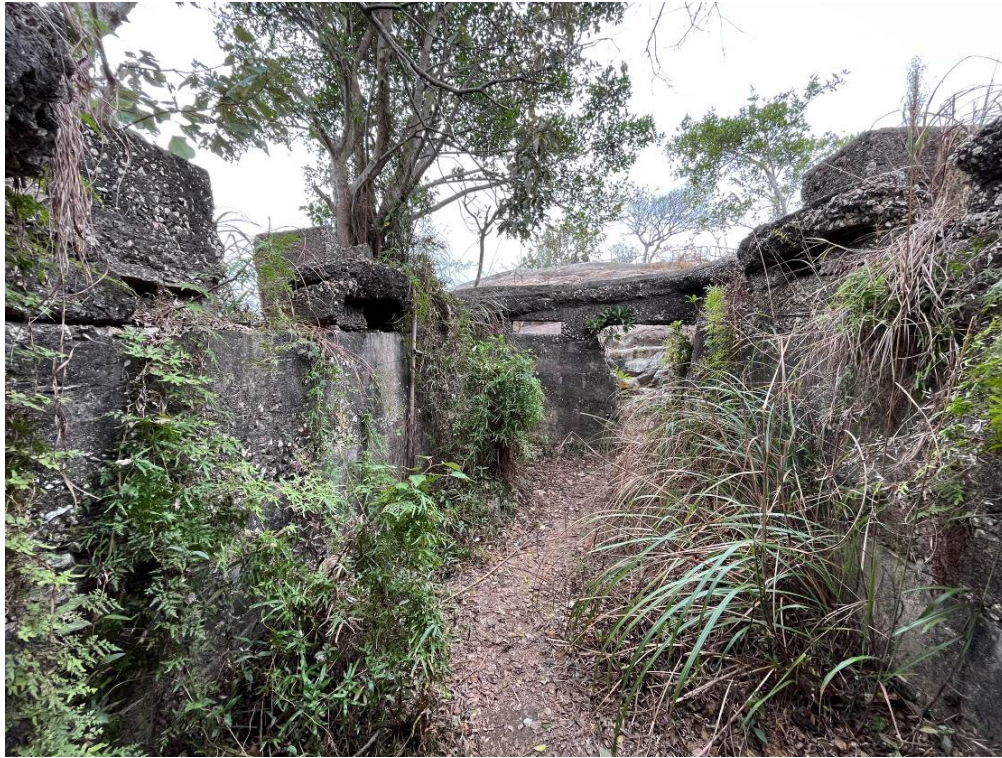
Plate 1.23. Concrete bunker within the redoubt.
