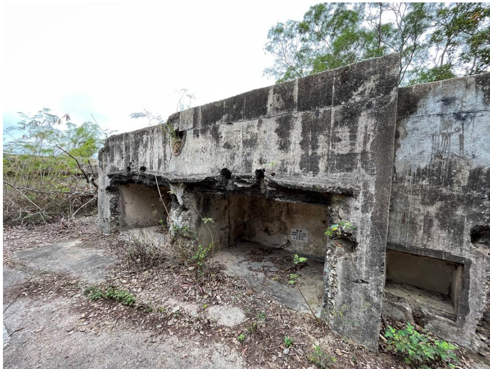
Plate 1.12. Storage space of the 9.8-inch gun emplacement.
