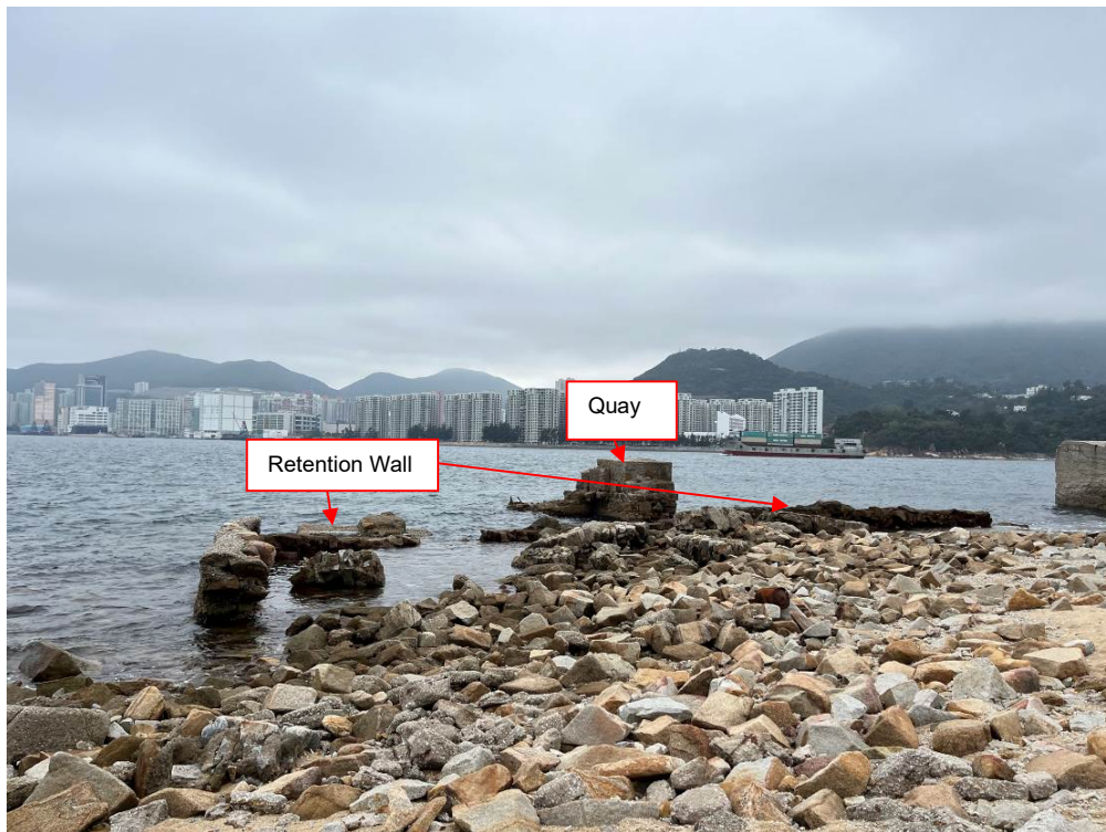
Plate 2.37. Remains of quay and retention walls in the south of the site.
