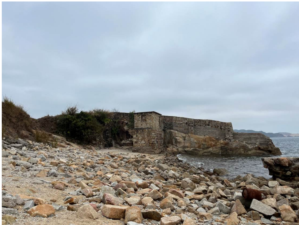
Plate 2.41. Seawall in the east of the site.
