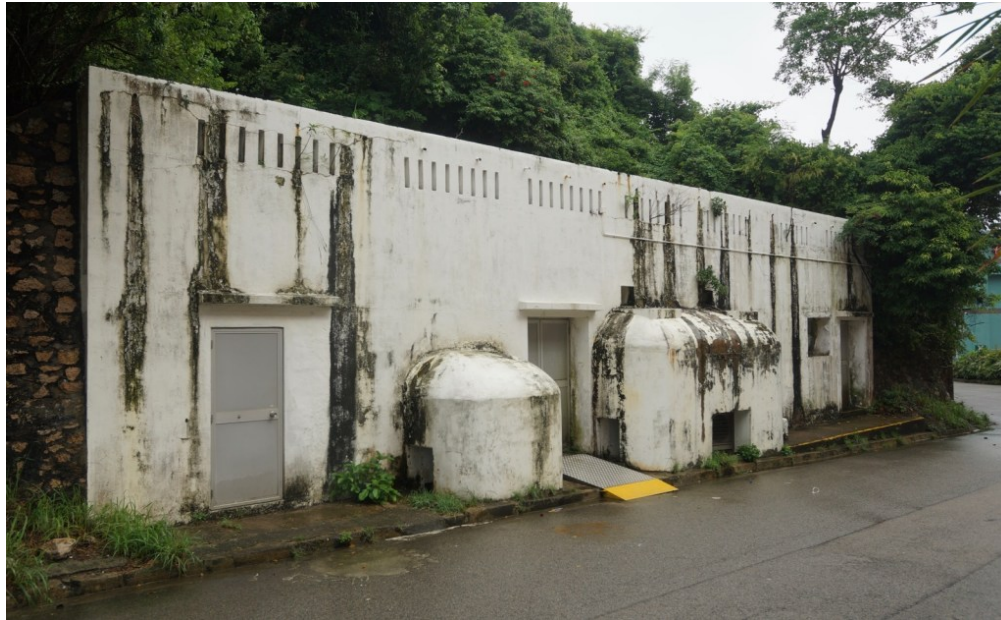
Plate 4.7. Bunker in Chung Hom Kok Battery (grade 2 historic building). The bunker has the same set of vertical rectangular slits along the upper edge of the front façade. Rectangular cuboids with rounded-corners can also be found.
