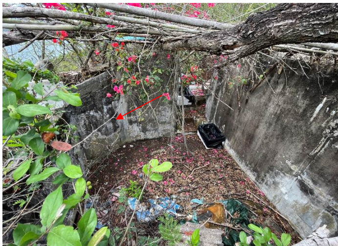
(Left) Plate 12.4. The interior of the pillbox, southern corner is chamfered (red arrow indicates).
