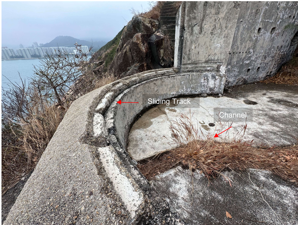
Plate 5.4. Sliding tracks could be found along the semi-circular front. A channel (probably gutter) was observed.
