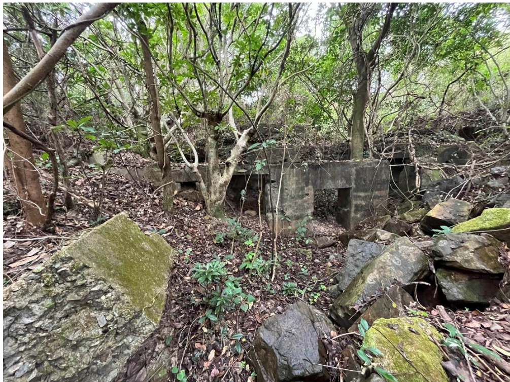
Plate 1.10. Collapsed bunkers of the Pottinger Battery.
