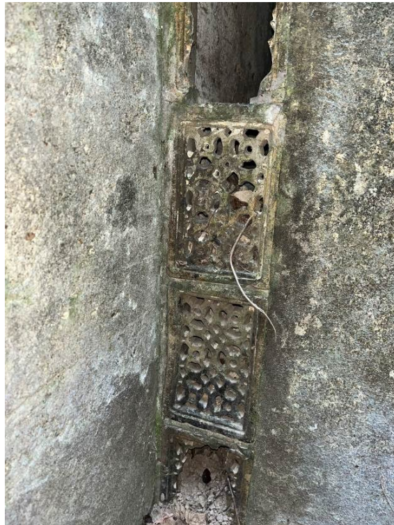
Plate 1.8. Ventilation tiles of Chinese coin patterns observed at the underground magazine.
