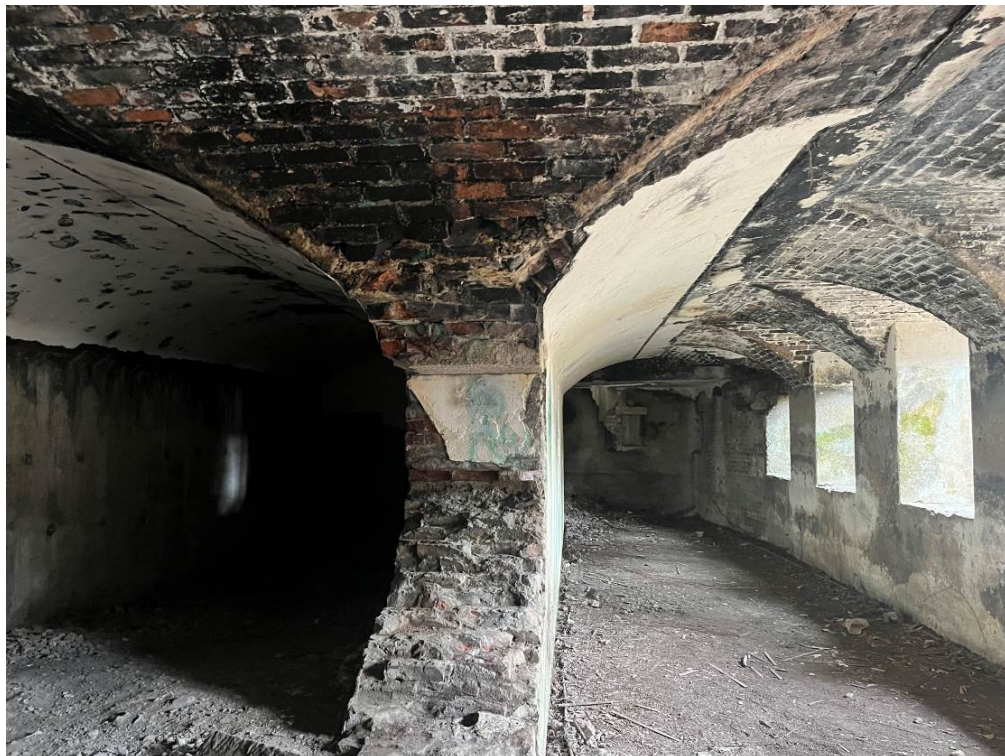
Plate 1.16. Interior of the underground magazine of the Gough Battery. Fine brickwork vaulting is observed.
