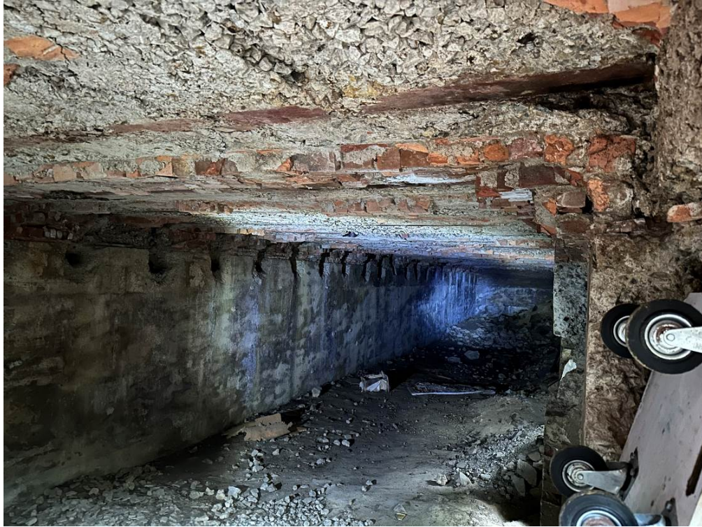
Plate 1.7. The main underground magazine of Pottinger Battery.
