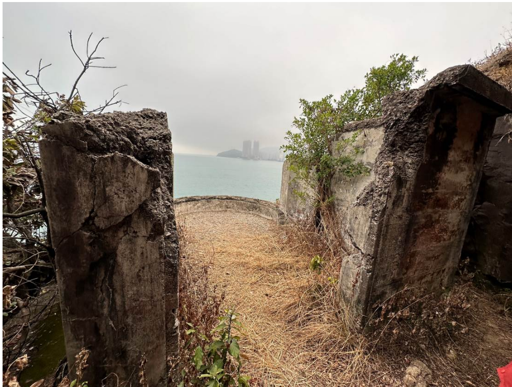
Plate 6.3. Rear elevation of the southern coastal searchlight emplacement.
