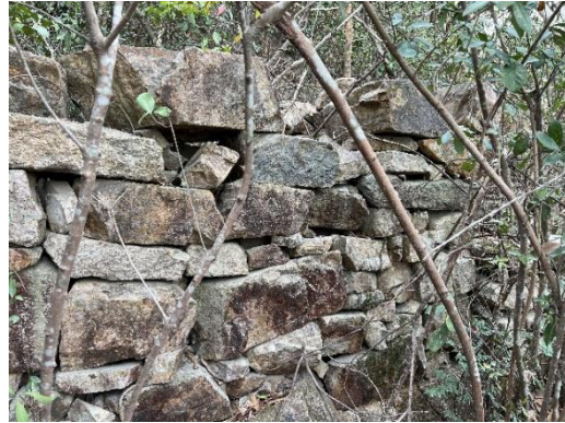
Plate 14. Retaining Wall built with granite slabs
