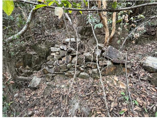
Plate 12. Front wall constructed of semi-dressed granite slab
