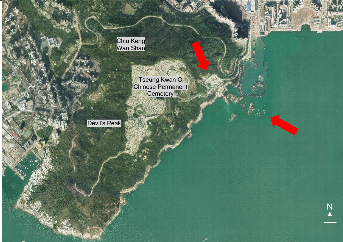
Plate 15. Aerial photo in 2019 showing the construction works for Tseung Kwan O-Lam Tin Tunnel.
