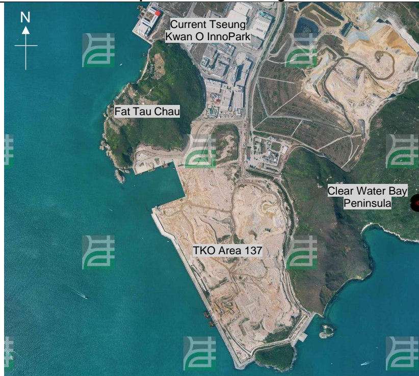
Plate 9. Aerial photo in 2005 showing TKO Area 137.
