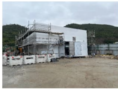
PHOTO 6804: TRANSFORMER ROOM IN CONSTRUCTION DATE TAKEN: 11 MARCH 2024
