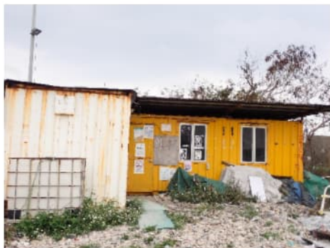
PHOTO 7888: WORKERS REST CONTAINERS DATE TAKEN: 19 FEBRUARY 2024
