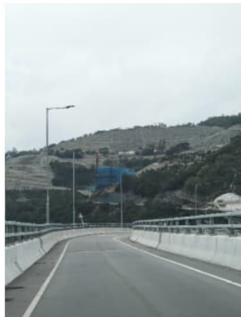
PHOTO 6037: TSEUNG KWAN O INTERCHANGE OF TSEUNG LAM HIGHWAY DATE TAKEN: 19 FEBRUARY 2024
