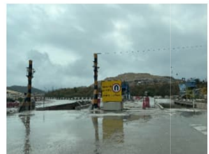
PHOTO 6567: WHEEL WASHING BAY DATE TAKEN: 22 FEBRUARY 2024
