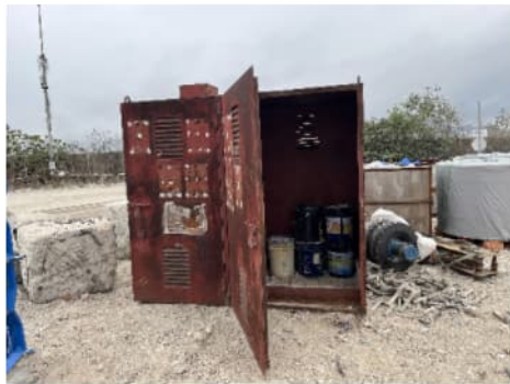
PHOTO 5302: CHEMICAL STORAGE CABINET DATE TAKEN: 19 FEBRUARY 2024
