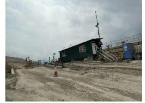
PHOTO 6244: WEIGHING POINT AND RECORDER HOUSE DATE TAKEN: 22 FEBRUARY 2024
