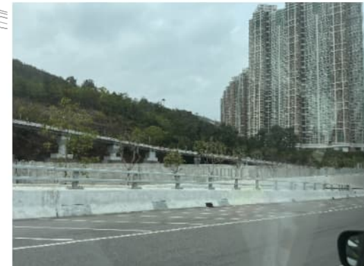
PHOTO 7887: ROAD P2 OF TSEUNG LAM HIGHWAY DATE TAKEN: 19 FEBRUARY 2024
