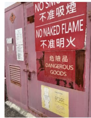
PHOTO 5709: DANGEROUS GOODS STORE DATE TAKEN: 22 FEBRUARY 2024
