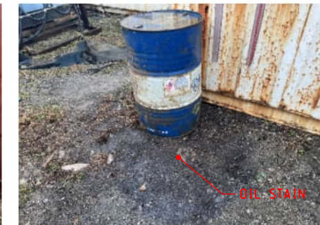
PHOTO 7010: OIL STAIN UNDERNEATH THE ENGINE OIL DRUM DATE TAKEN: 11 MARCH 2024
