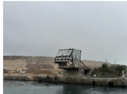
PHOTO 9893: TIPPING HALL DATE TAKEN: 20 MARCH 2024
