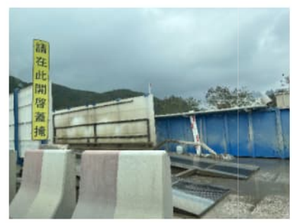
PHOTO 6521: WASH HOUSE DATE TAKEN: 22 FEBRUARY 2024
