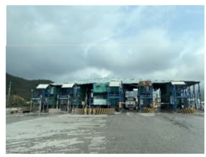
PHOTO 6451: COMBINED RECEPTION AND EXIT OFFICES DATE TAKEN: 22 FEBRUARY 2024
