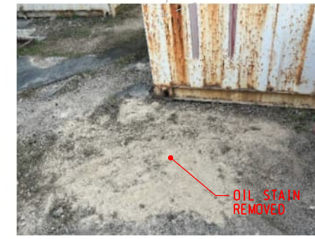
PHOTO 0074: OIL STAIN REMOVED DATE TAKEN: 26 MARCH 2024
