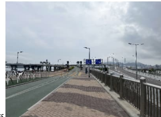
PHOTO 5518: PEDESTRIAN ROAD AND CYCLING TRACK DATE TAKEN: 19 FEBRUARY 2024
