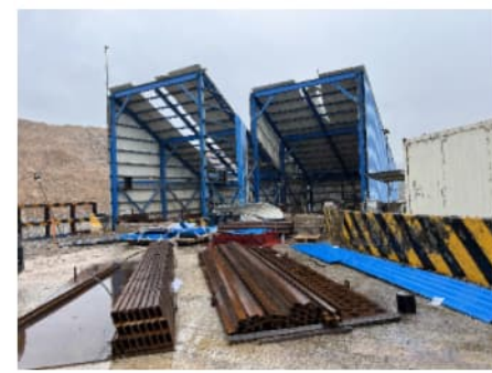
PHOTO 7042: TIPPING HALL DATE TAKEN: 11 MARCH 2024
