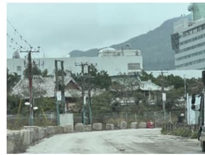
PHOTO 5450: ACCESS ROAD DATE TAKEN: 19 FEBRUARY 2024
