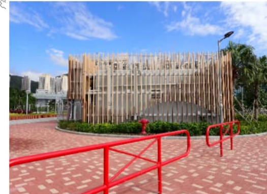
PHOTO 9406: ROAD P2 STORMWATER PLANT ROOM SUBSTATION DATE TAKEN: 16 OCTOBER 2024
