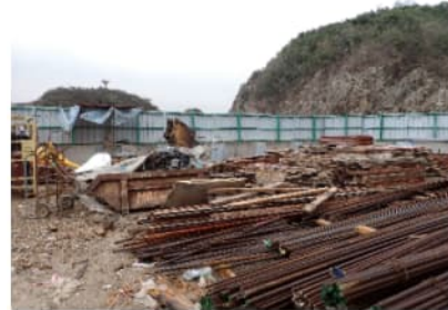
PHOTO 8529: CONSTRUCTION MATERIAL STORAGE AREA DATE TAKEN: 11 MARCH 2024
