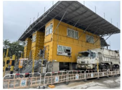
PHOTO 7708: COMBINED RECEPTION AND EXIT OFFICE DATE TAKEN: 19 FEBRUARY 2024
