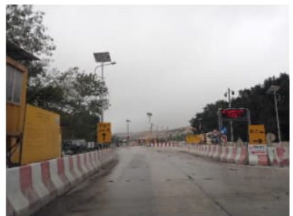
PHOTO 7928: ACCESS ROAD DATE TAKEN: 22 FEBRUARY 2024
