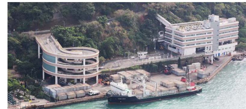
| Island West Transfer Station
