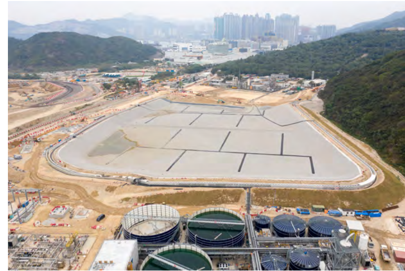
Construction of the SENT Landfill extension in progress
