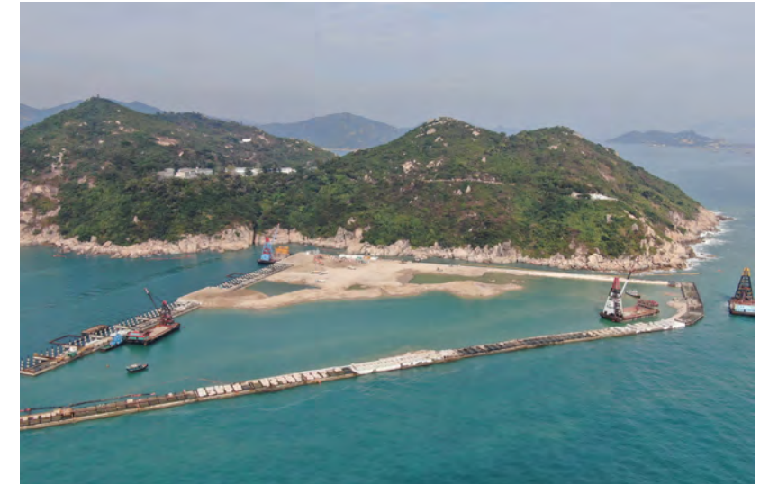
| Reclamation of artificial island for I-PARK in progress (December 2020)
