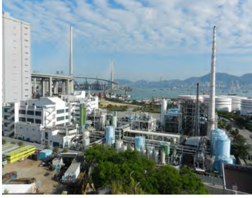
Chemical Waste Treatment Centre
