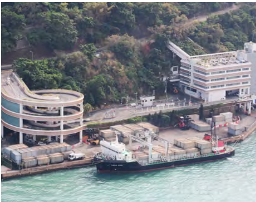
Island West Transfer Station
