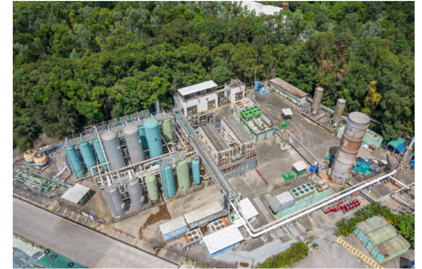
Landfill Gas Utilisation Plant at the NENT Landfill
